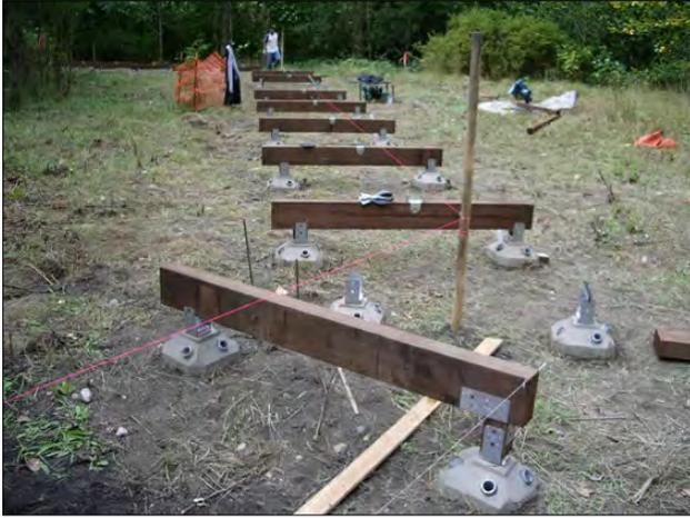
**FIGURE 4.8.3 - FOOTBRIDGE WITH MINIMAL EXCAVATION FOUNDATION**
