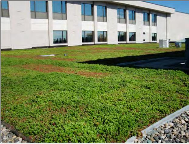
**FIGURE 4.7.1 - VEGETATED ROOF – EXTENSIVE DESIGN**
