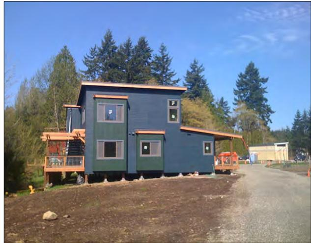
**FIGURE 4.8.1 - USE OF MINIMAL EXCAVATION FOUNDATIONS FOR RESIDENTIAL DWELLING**
