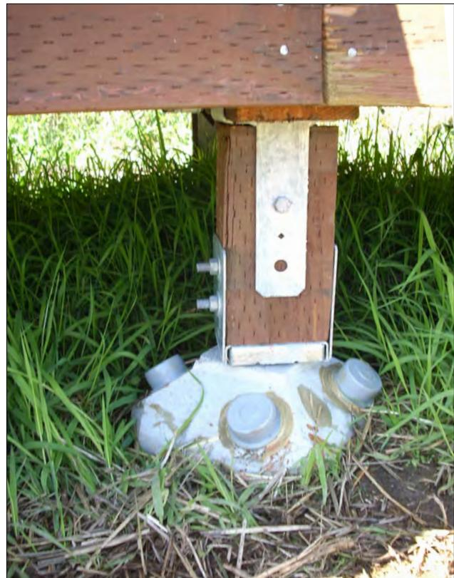
**FIGURE 4.8.5 - PIER TYPE MINIMAL EXCAVATION FOUNDATION**
