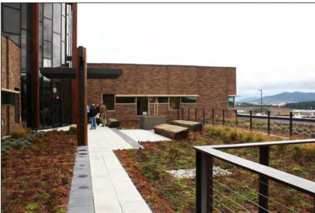
**FIGURE 4.7.2 - VEGETATED ROOF – INTENSIVE DESIGN**
