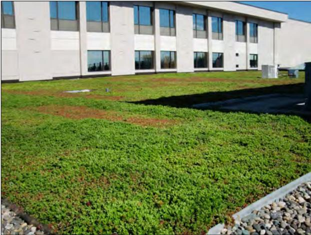
**FIGURE 4.7.1 - VEGETATED ROOF – EXTENSIVE DESIGN**
