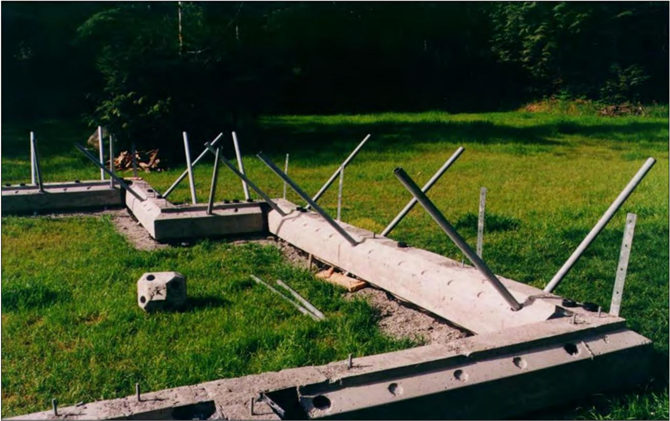
FIGURE 4.8.6 - WALL TYPE MINIMAL EXCAVATION FOUNDATION
