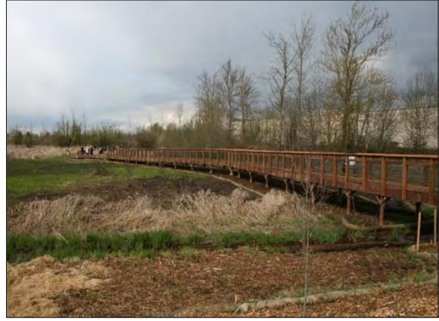
**FIGURE 4.8.4 - FOOTBRIDGE WITH MINIMAL EXCAVATION FOUNDATION**
