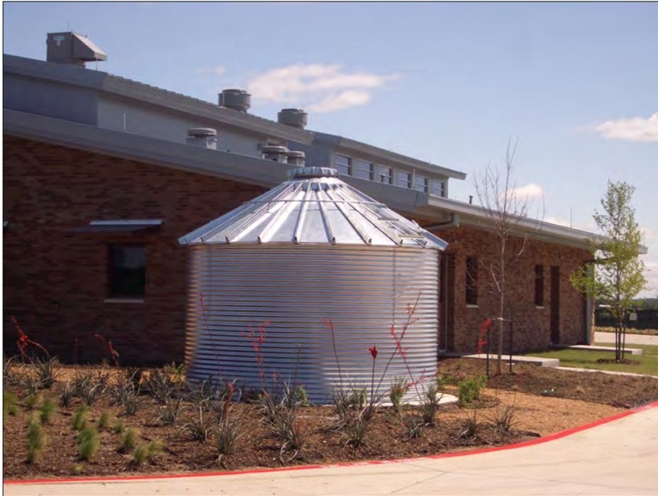
**FIGURE 4.9.3 - CISTERN USED TO MEET NON-POTABLE WATER NEEDS**
