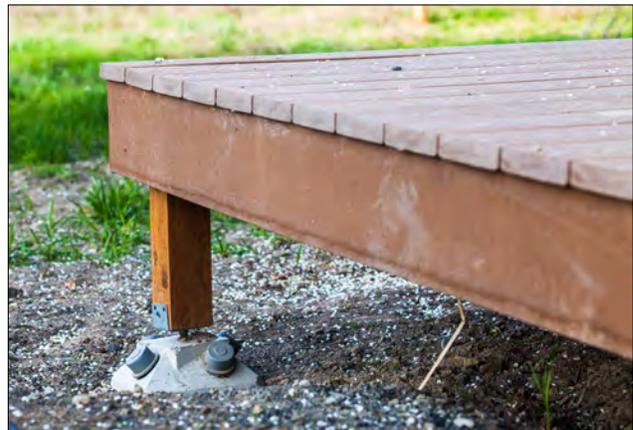
**FIGURE 4.8.2 - USE OF MINIMAL EXCAVATION FOUNDATIONS FOR ACCESSORY STRUCTURES**
