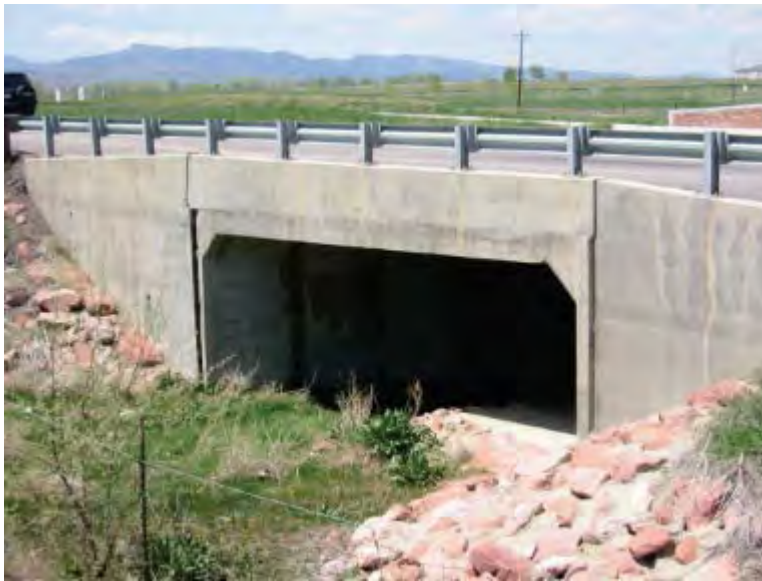
Figure 3-2 Concrete Box Culvert
