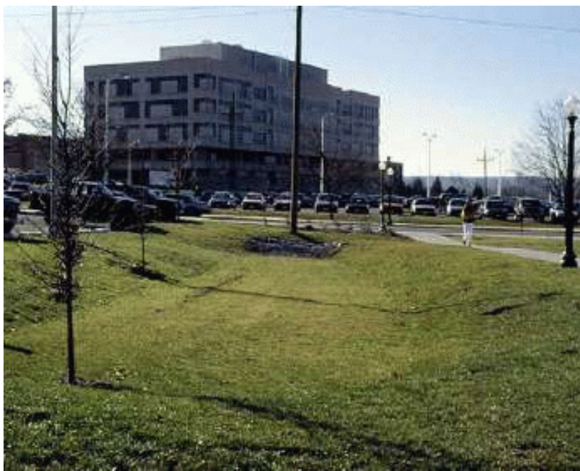
Figure 6-2 Grass Swale with Check Dam (VA DEC, 1999)
