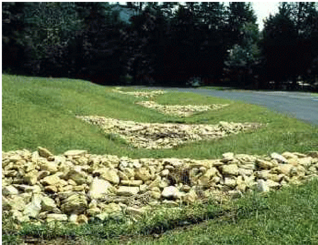
Figure 6-3 Grass Swale with Check Dams (VA DEC, 1999)
