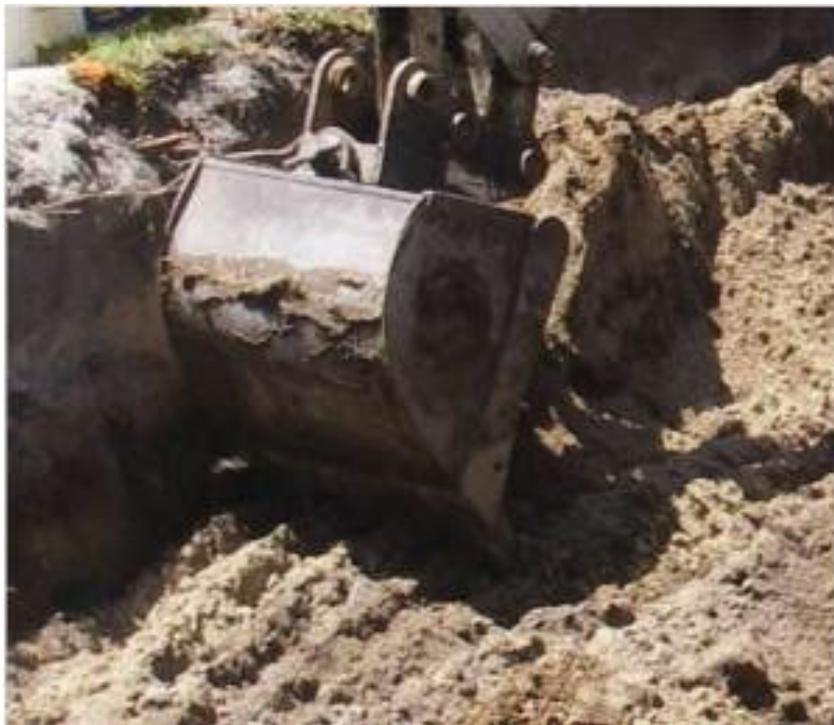
Figure 60. For infiltrating practices, mitigate subsoil compaction by ripping grade to a depth of 12 inches.
