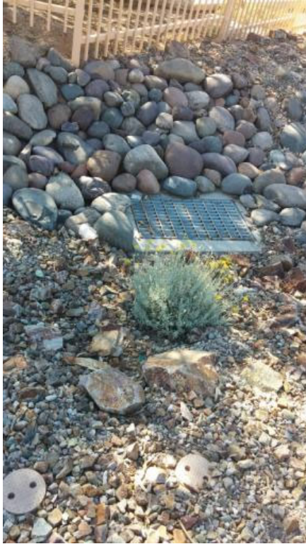
Figure 54. An outlet connected directly to a storm drain at the downstream end of a stormwater harvesting basin.
