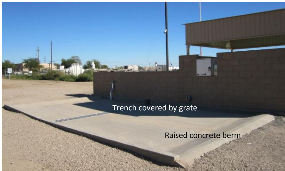
Figure 24. Containment structure for vehicle washing set in gravel.
