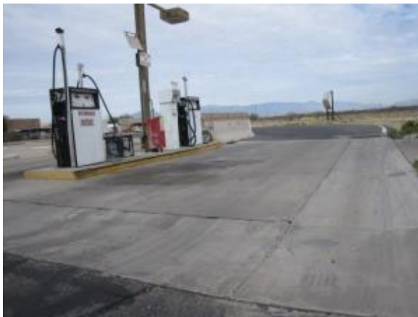
Figure 25. Fuel station with sloped gutter leading to a sump.
