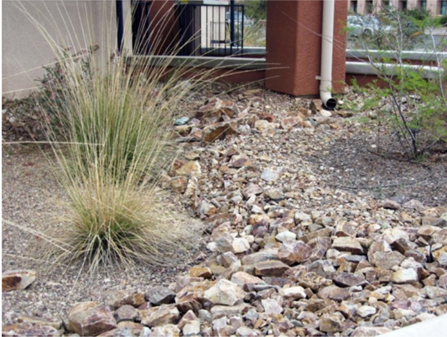
Figure 17. Downspout flow disconnected from impervious drive surfaces; directed to a pervious area.
