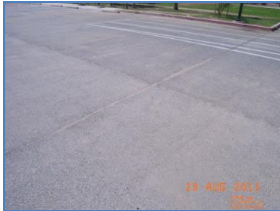
Figure 46. Example pervious concrete installation (left). Typical pervious concrete detail (right).
