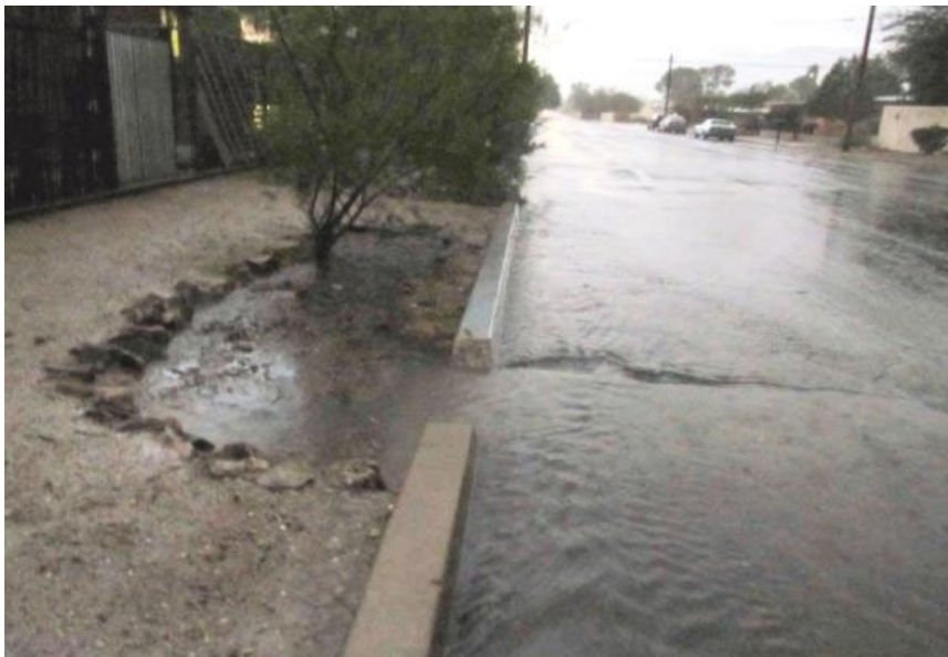
Figure 53. The inlet to this stormwater harvesting basin also functions as an outlet.
