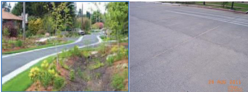
Figure 18. LID street design (left), permeable parking lot (right).
