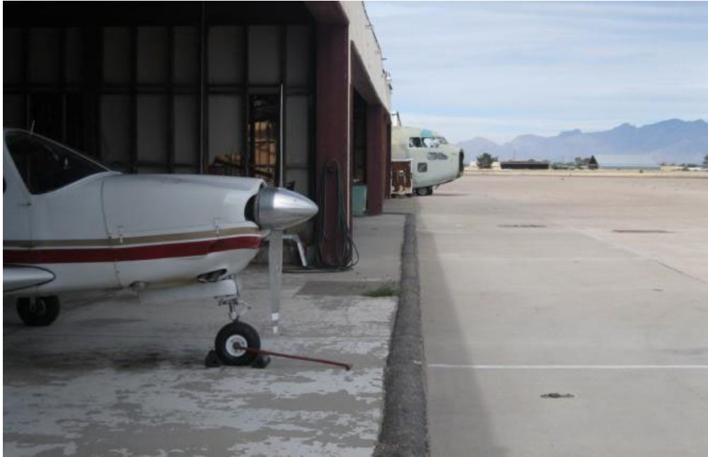
Figure 23. Maintenance bay with covering and low level berm to prevent run-on.
