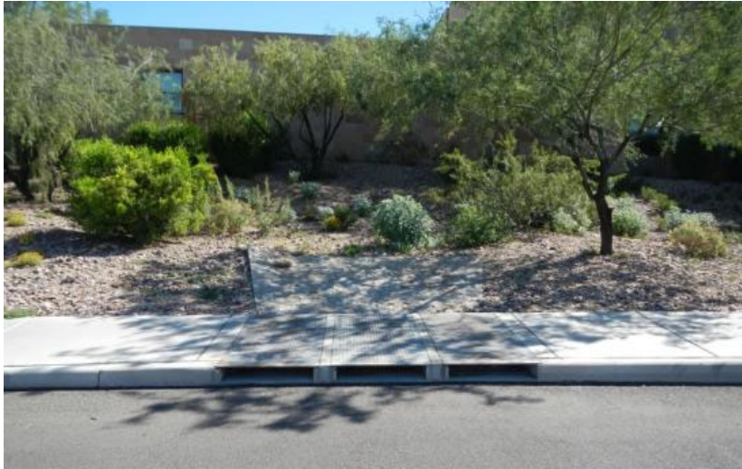
Figure 55. This figure shows the downstream outlet of a stormwater harvesting basin that discharges to the street once the basin is at capacity.
