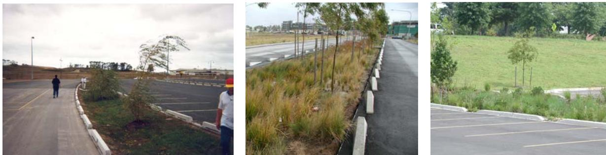
**Figure 7.12. Photograph of different arrangements of kerbs with breaks to distribute inflows**
