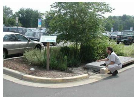
*Bioretention basins are applicable at a range of scales and can be integrated with an urban landscape*
