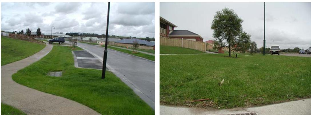
**Figure 7.17. Similar buffer swale system for conveying runoff**
