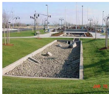
*Sand filters can be installed above or below ground*
