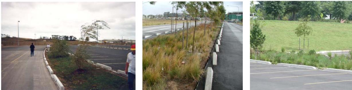
**Figure 4.9. Photograph of kerbs with breaks to distribute inflows**
