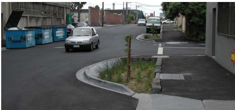
**Figure 5.7.** Retrofitted Bioretention System in a street
