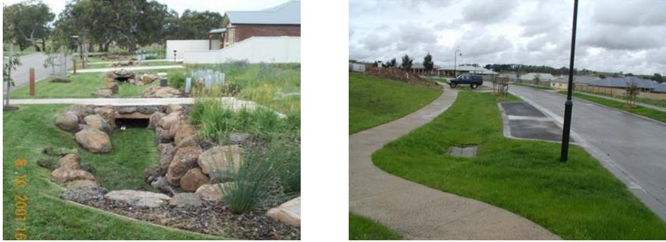
**Figure 7.3. Elevated and at-grade driveway crossings across swales**
