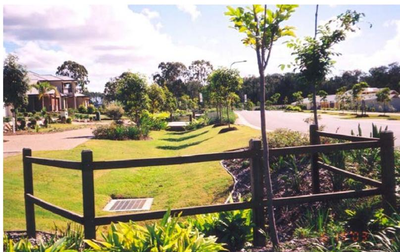
Figure 4.12. Photograph of bioretention swale
