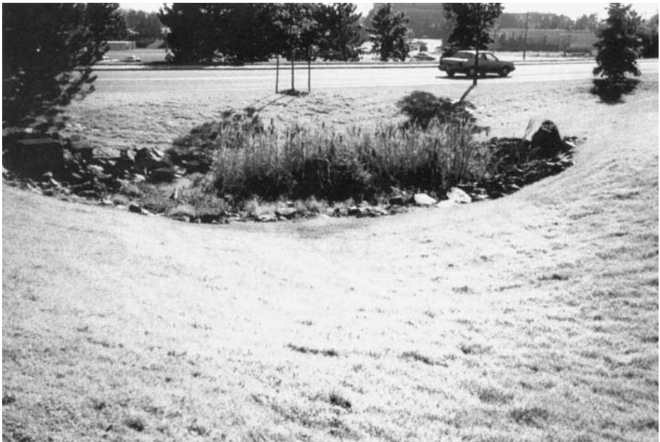
FIGURE 8.6 Infiltration and retention system.
