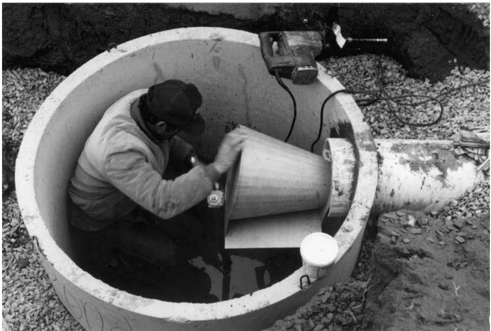
FIGURE 18.30 6-Inch Type “C” Conical Reg-U-Flow Vortex Valve. Installed in a 4-ft diameter catchbasin. This unit was supplied with a sleeve pipe which was inserted into the outlet pipe and sealed by 2 neoprene rubber “O” rings. The consultant on this project wished to maintain a silt trap so the control unit was mounted 3-feet above the base of the chamber with an additional support member to anchor the base of the cone. (From HydroInternational, PLC)
