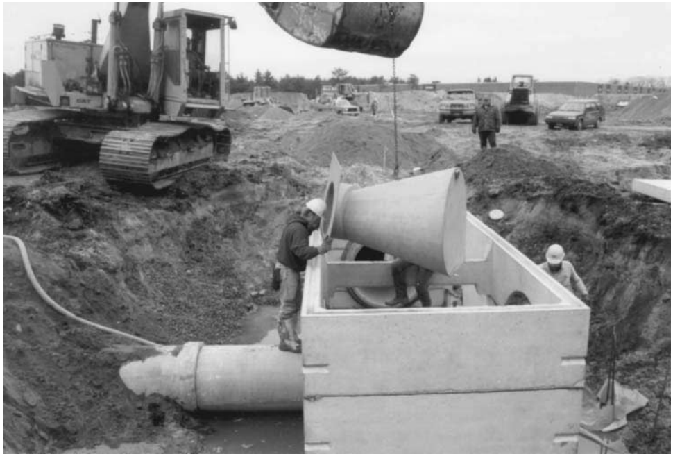
FIGURE 18.31 Type “C” Reg-U-Flo Vortex Valve. A 22-inch Type “C” Reg-U-Flo Vortex Valve discharging 15 cfs (425 l/s), installed at the Eastern Mall Office Park project in South Portland, Maine. This photograph shows the valve being lowered into place in the precast concrete control chamber. This stormwater management project was designed by H.I.L. Technology, Inc. By storing the 2-year storm within the pipes and manholes and the 25-year storm on the parking lots, the developer was able to avoid the construction of a detention pond which would have required the purchase of additional land. (From HydroInternational, PLC)
