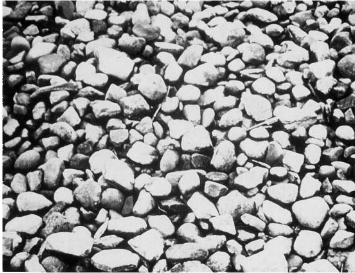
FIGURE 16.7 Gravel channel lining.
