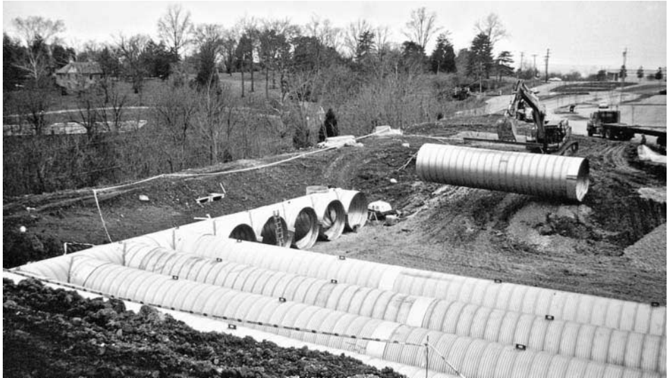
FIGURE 13.1 108" diameter detention system.
