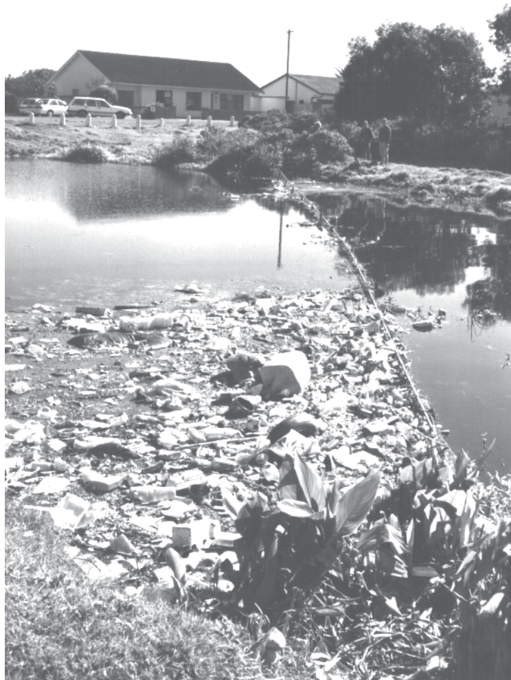
FIGURE 19.18 View of litter trapped behind a fence strung across a river.
