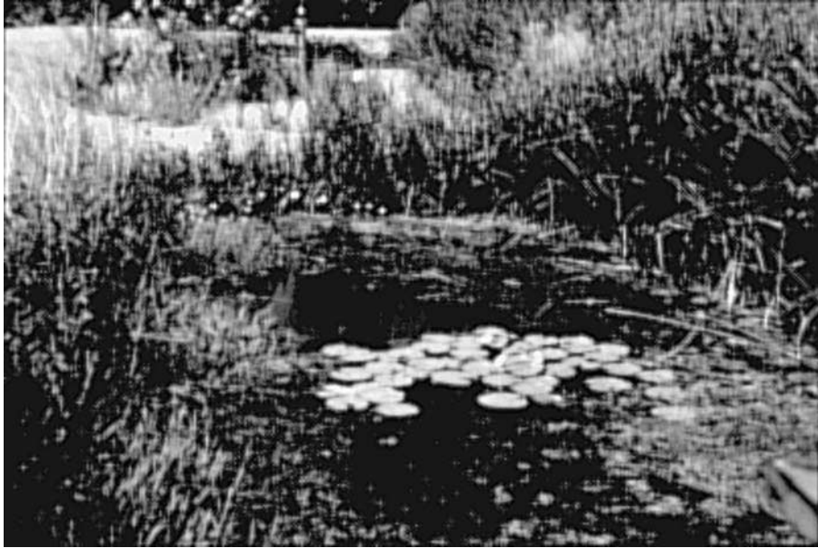
FIGURE 10.8 Outlet deep-zone to permit even discharge of wetland waters planted with floating aquatic plants to reduce sunlight transmission as a means of controlling algal development in an open-water zone.
