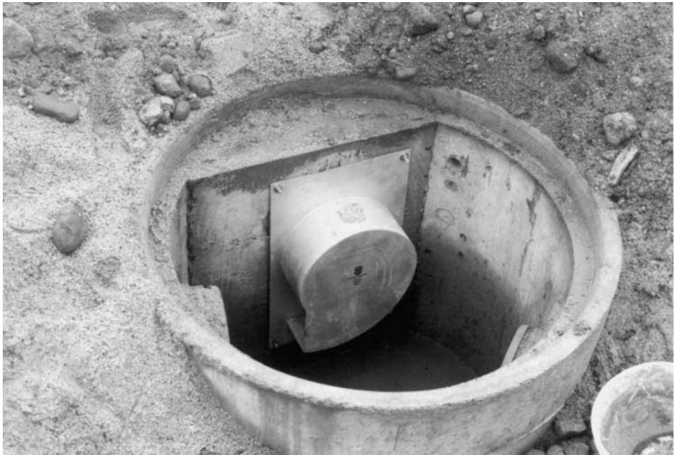
FIGURE 18.29 Plate mounted Type “SH” Vortex Valve. Design discharge of 0.42 cfs (12 l/s) under a 5-foot head, City of Portland, Maine. The “SH” unit was installed in a 4-ft. diameter manhole. Intake to the unit is on the bottom left. This unit is plate mounted as the outlet pipe is larger than the casing of the control unit. Normally, this type of unit is fixed using 3 lugs and anchor bolts or a push-fit spigot/sleeve arrangement. (From HydroInternational, PLC)
