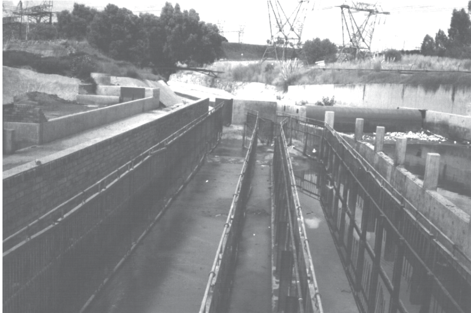
FIGURE 19.17 View of the Robinson Canal screens after cleaning. The hydraulically operated sluice gate is clearly visible on the top right-hand side of the picture.
