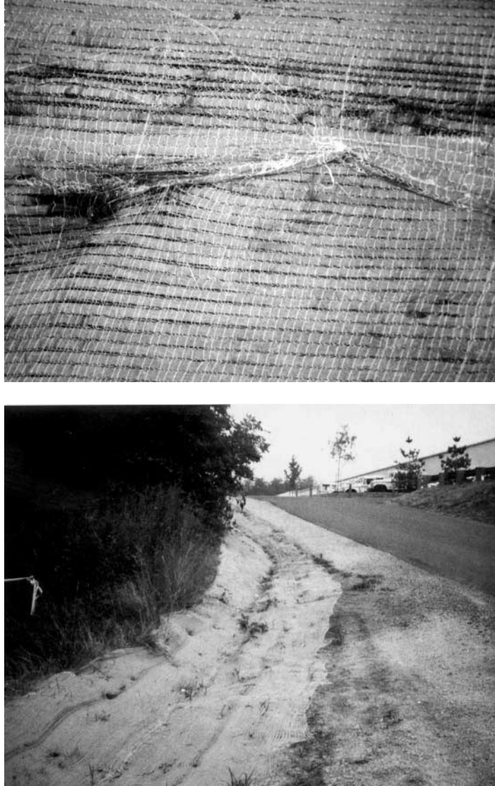
FIGURE 16.9 Woven-paper net channel lining.
