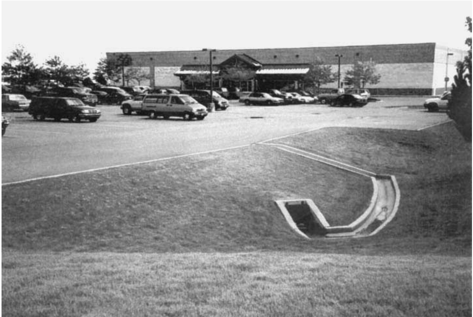
FIGURE 8.5 Detention system in parking area.
