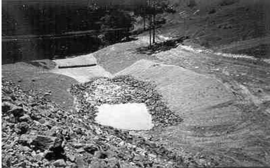
FIGURE 17.7 Riprap application. (From IECA, 1998)
