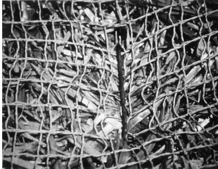
FIGURE 16.12 Straw with net channel lining.
