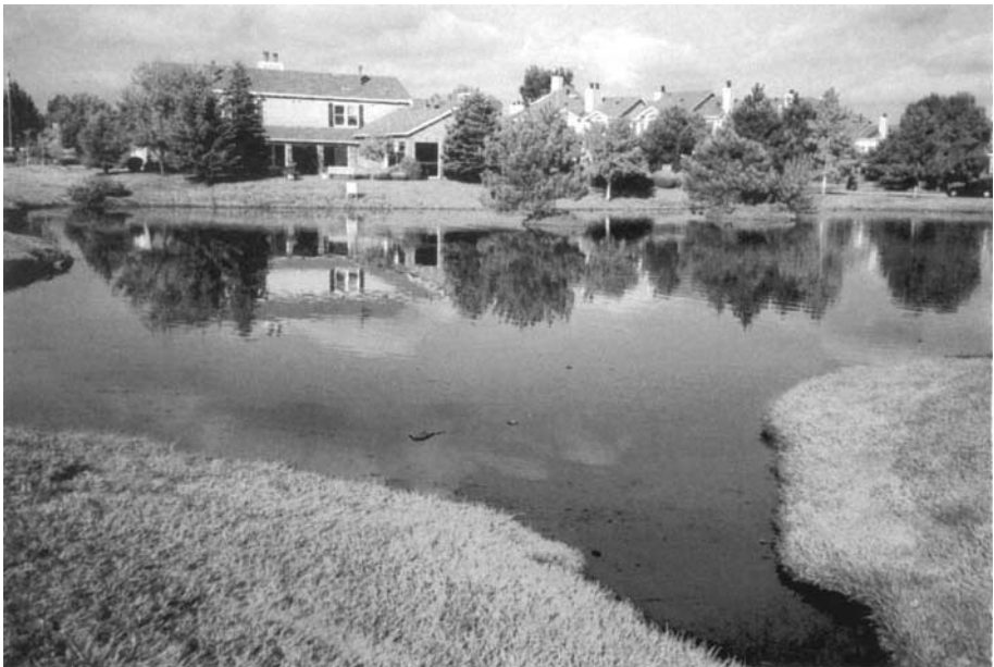
FIGURE 9.7 Large infiltration basin with 12- to 18-inch shallow depth.
