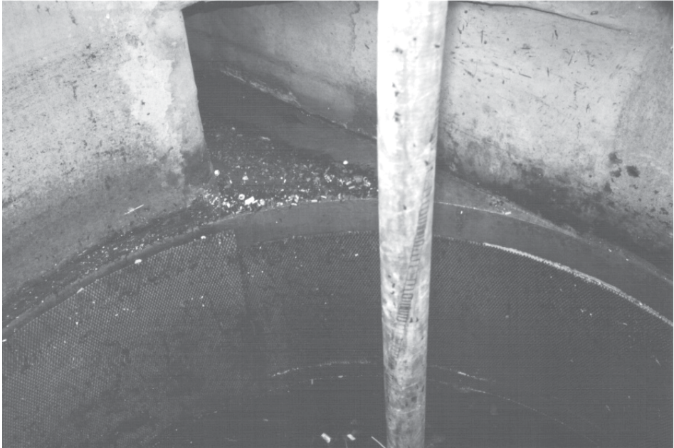
FIGURE 19.11 View of the inside of a CDS device. The unit is being drained for cleaning. The inlet culvert and the screen are clearly visible.
