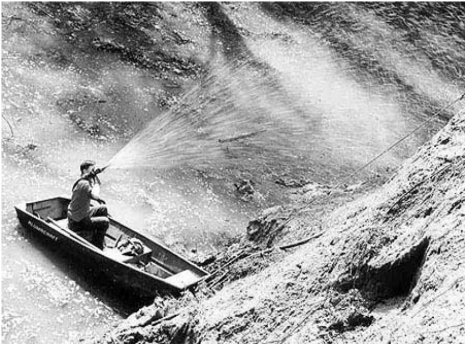
FIGURE 17.2 Hydraulic seeding. (From IECA, 1998)
