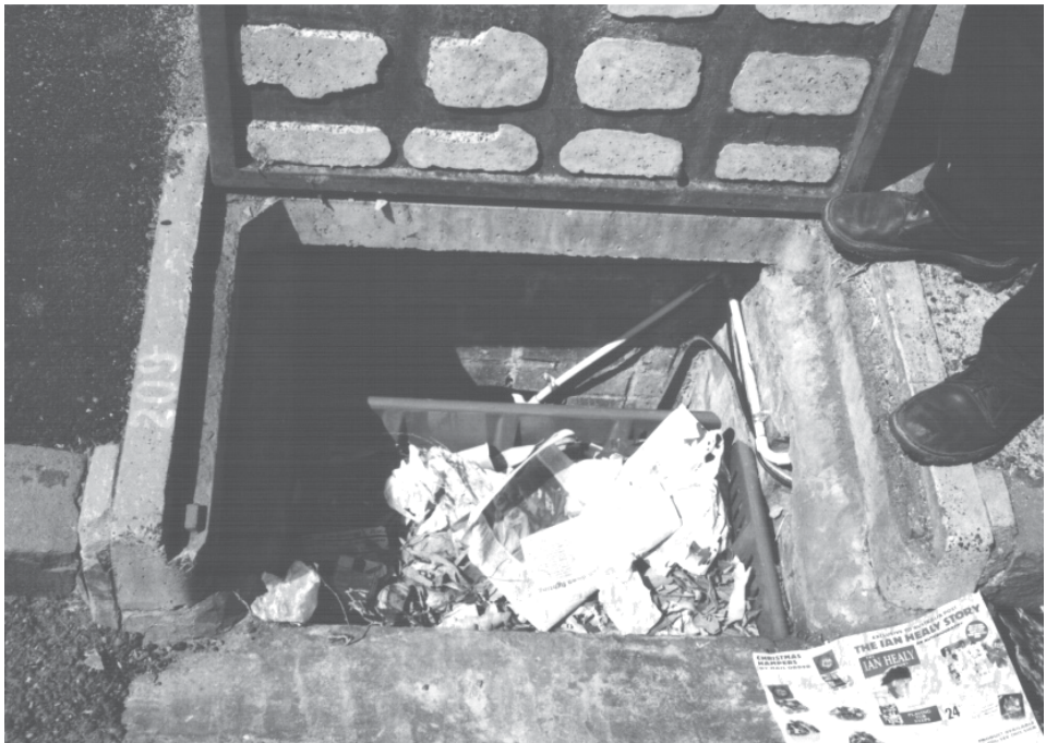
FIGURE 19.5 View of a typical side-entry catchpit trap.
