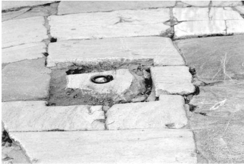
FIGURE 1.6 (Continued) (c) Cover to underground drainage.
