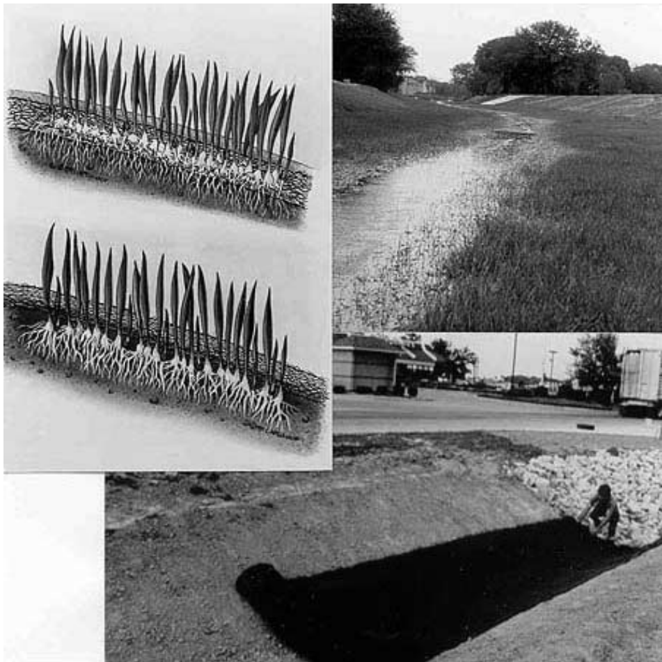
FIGURE 17.3 Temporary seeding applications. (From IECA, 1998)
