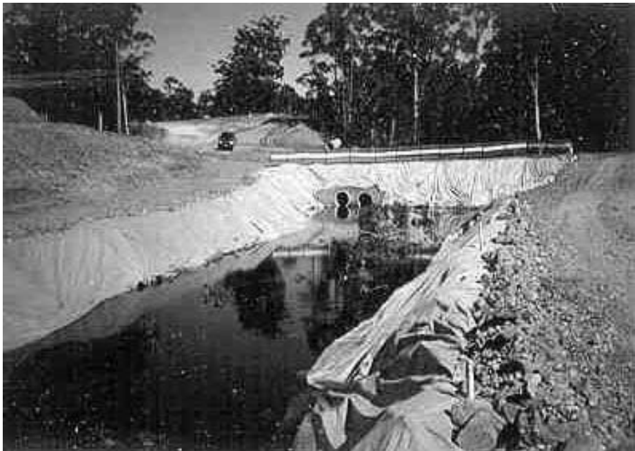
FIGURE 17.4 A typical geotextile application. (From IECA, 1998)
