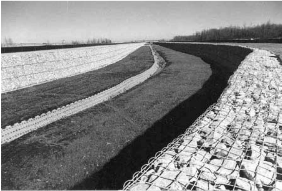
FIGURE 17.8 Grass-lined channel with gabion basket. (From IECA, 1998)
