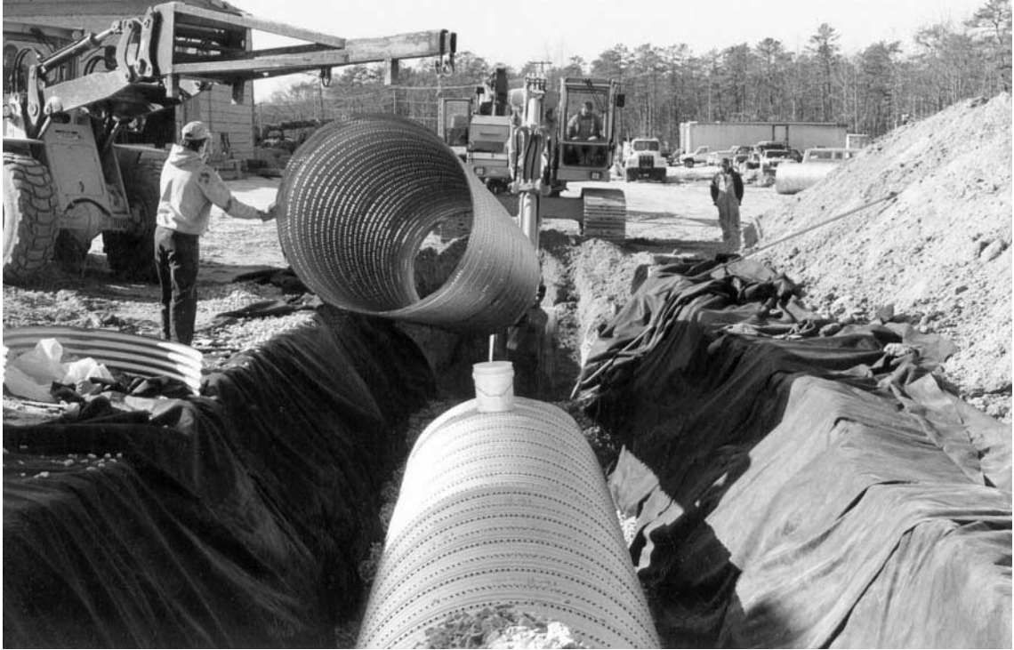
FIGURE 13.2 60" perforated CSP infiltration system.
