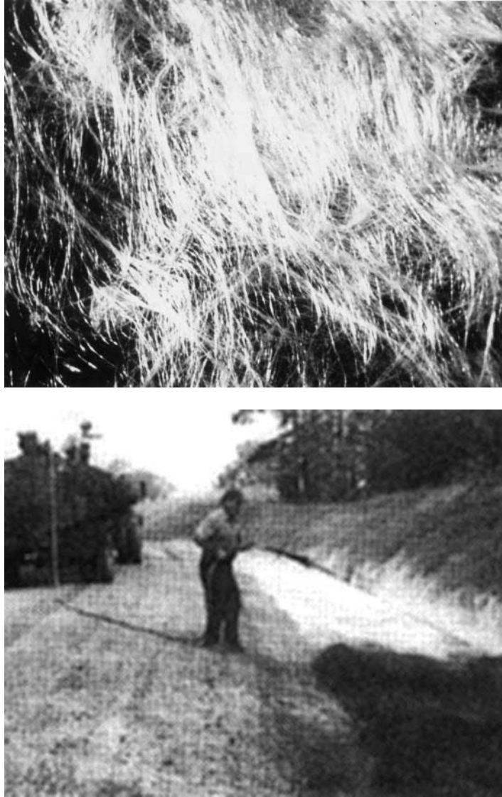
FIGURE 16.13 Fiberglass roving channel lining.
