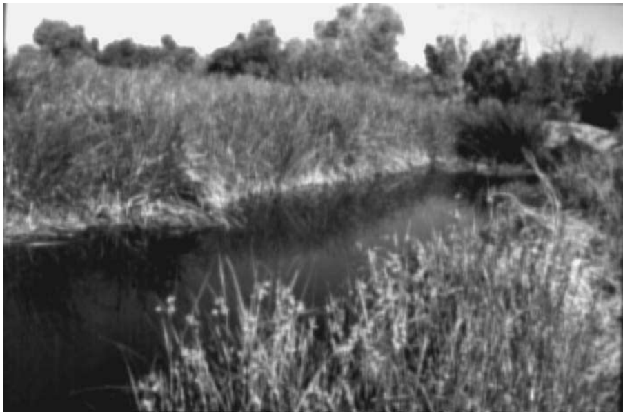
FIGURE 10.10 Internal deep-zone provides an open water surface for gas exchange and waterfowl, while at the same time enhancing mixing and mitigating short-circuiting in upstream shallow emergent marsh zones.
