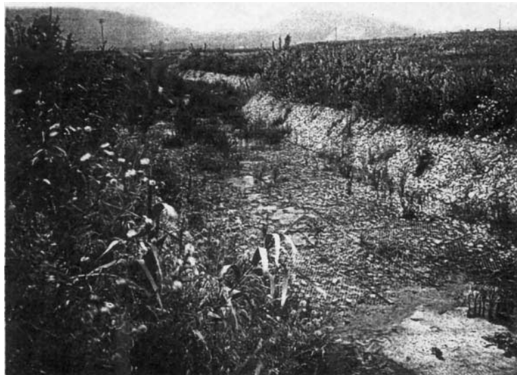
FIGURE 16.6 Wire-enclosed stone channel lining.
