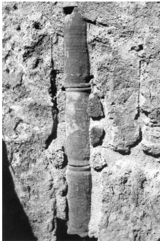
FIGURE 1.3 Tile for roof runoff that connects to cistern. (a) Tile. (Photos by L. W. Mays)
