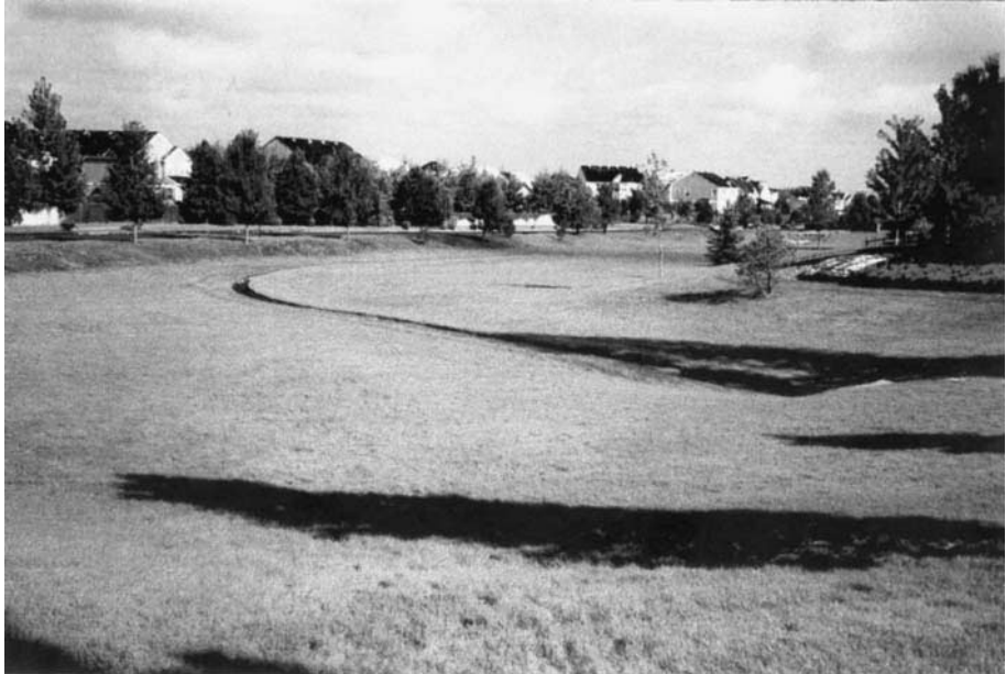
FIGURE 8.3 Example of channel detention on floodplain.
