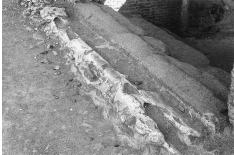
FIGURE 1.2 (Continued) (c) Drainage pipe along street.
