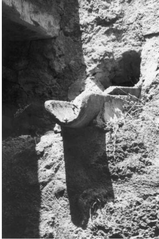
FIGURE 1.3 (Continued) (c) Gutter for roof runoff.
