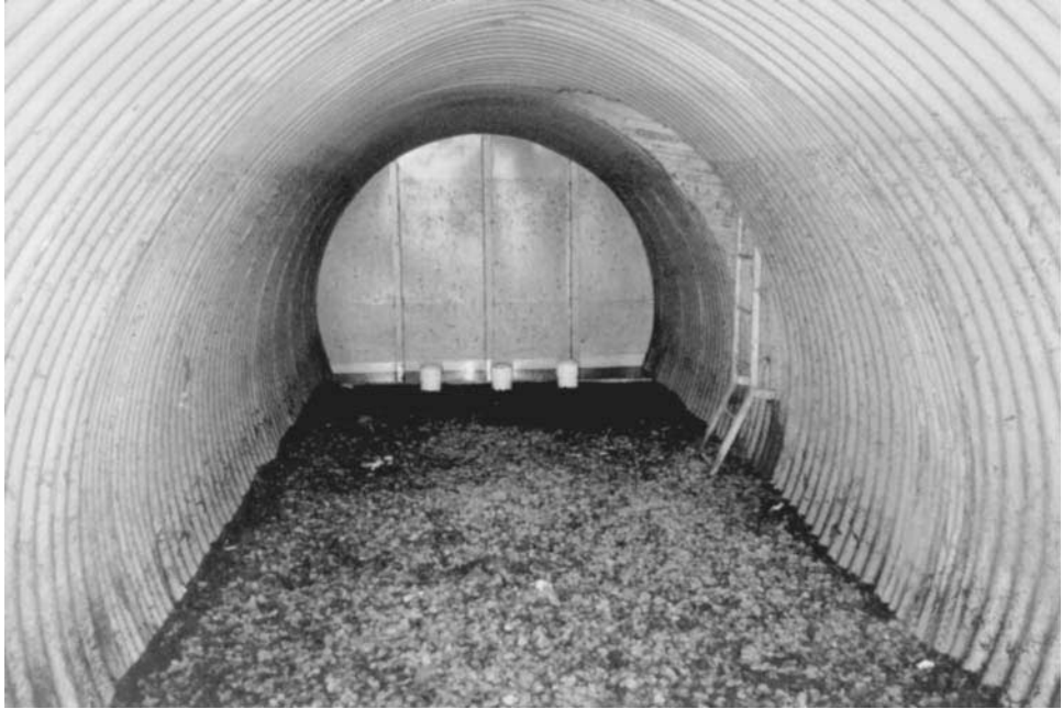
FIGURE 13.4 120" CSP sand filter.
