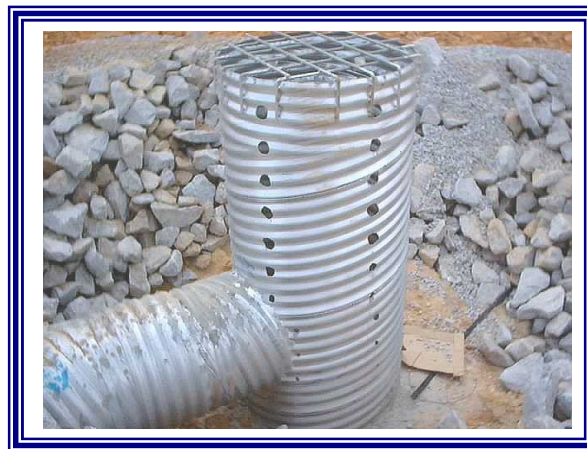
Temporary Sediment Basin Perforated Riser
