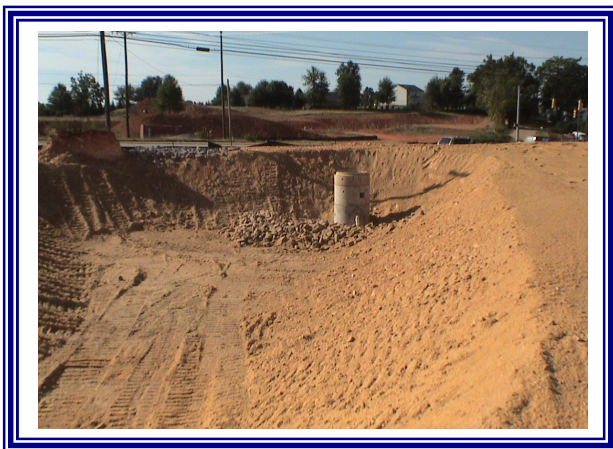
Temporary Sediment Basin
