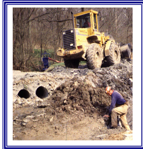
Temporary Stream Crossing
