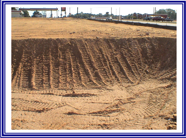
Surface Roughening (Tracking)
