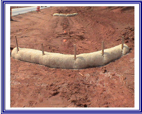
Sediment Tube Check Dam
