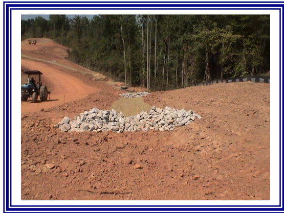
Rock Check Dam
