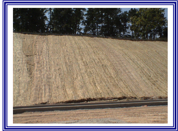
ECB Slope Application
