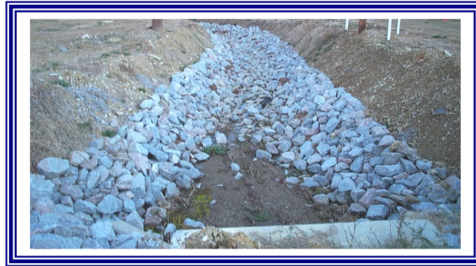
Riprap Lined Channel
