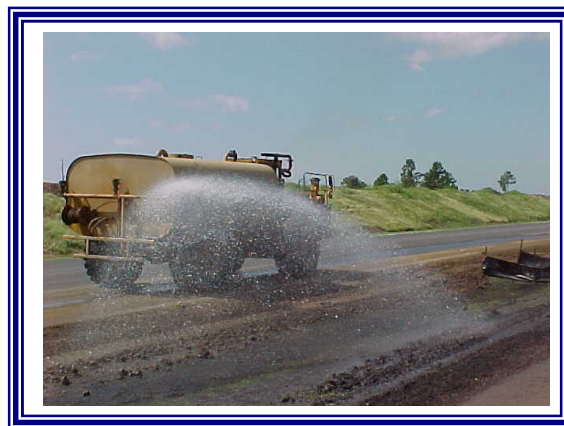
Dust Control by Sprinkling Water
