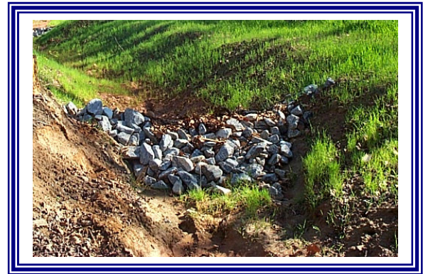
Rock Check Dam
