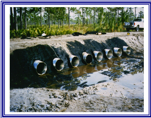
Temporary Stream Crossing
