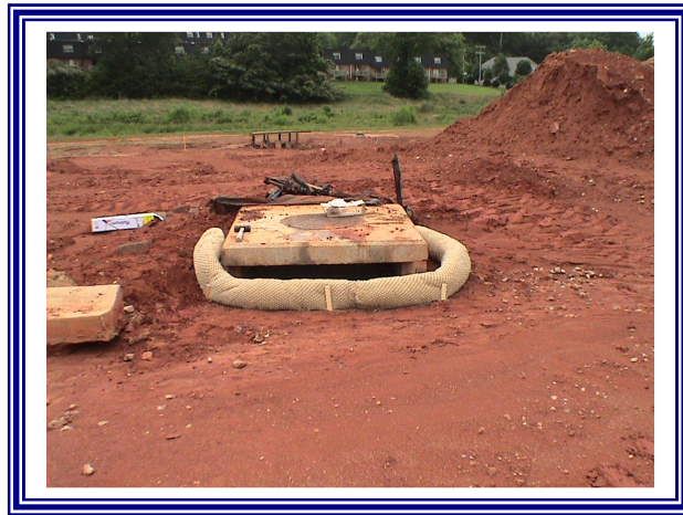
Sediment Tube Inlet Protection
