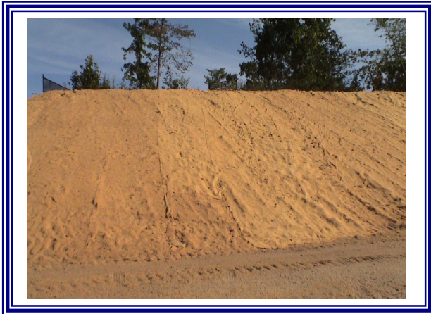
ECB Slope Application
