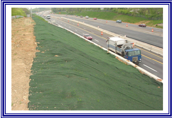
TRM Slope Application
