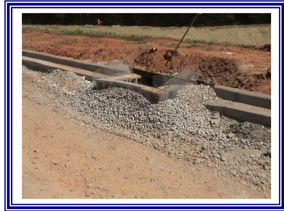
Block and Gravel Inlet Protection
