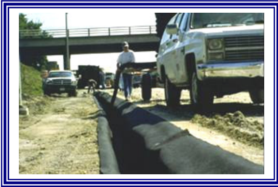
Subsurface Drain
