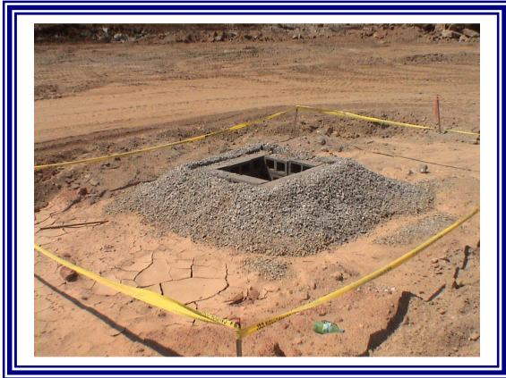
Block and Gravel Inlet Protection
