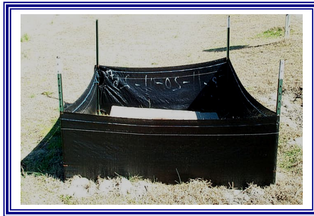
Filter Fabric Inlet Protection
