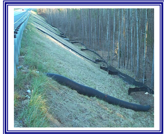
Pipe Slope Drain
