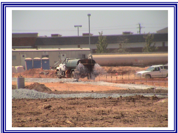
Dust Control by Sprinkling Water
