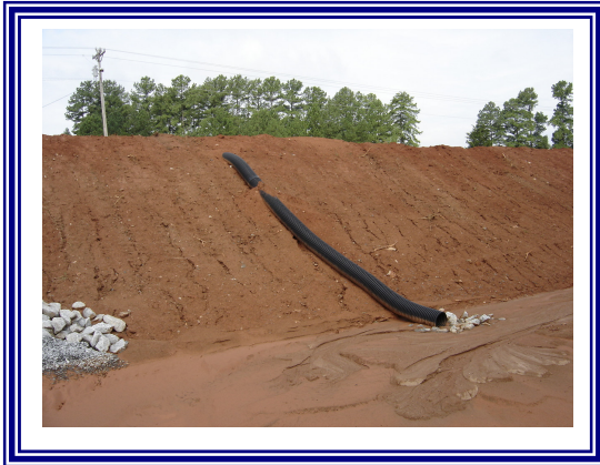
Pipe Slope Drain
