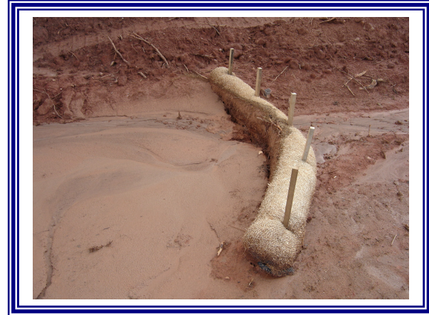
Sediment Tube Check Dam
