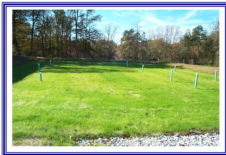
Bioretention Area with uncut clean outs
