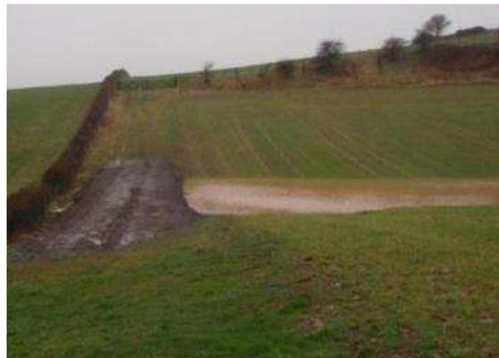
*Figure 19 – Field bund, acting as a raised access track, storing overland flow during heavy rain*
