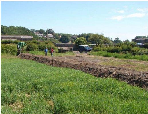
*Figure 18 – Bund being constructed across primary flow pathway*
