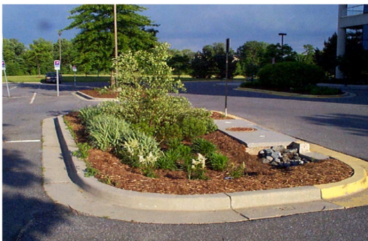
Figure 12-1 Bioretention in Parking Lot Island
