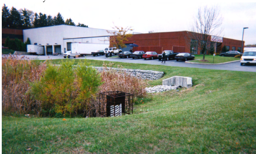
Figure 17-1 Dry Extended Detention Basin with Shallow Marsh
