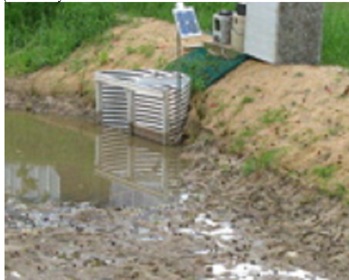
Figure 9-9 Outlet Structure With Flashboard Riser for Maintenance (Wetland Partially Drained) (Courtesy of Sharon Schulze, NC State Science House)
