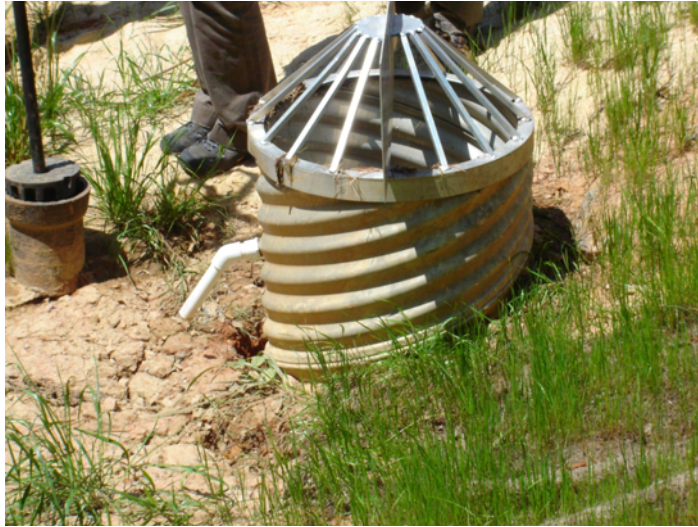
Figure 9-10 Outlet Structure With Down-Turned Drawdown Orifice
