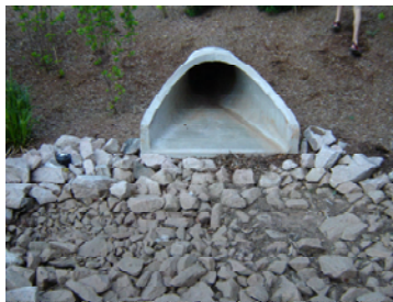
Figure 12-2b Bioretention Cell with Pretreatment: Forebay
