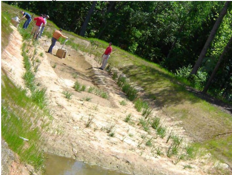
Figure 9-5 A Wetland Design Should Not Be Located Above the Water Table
