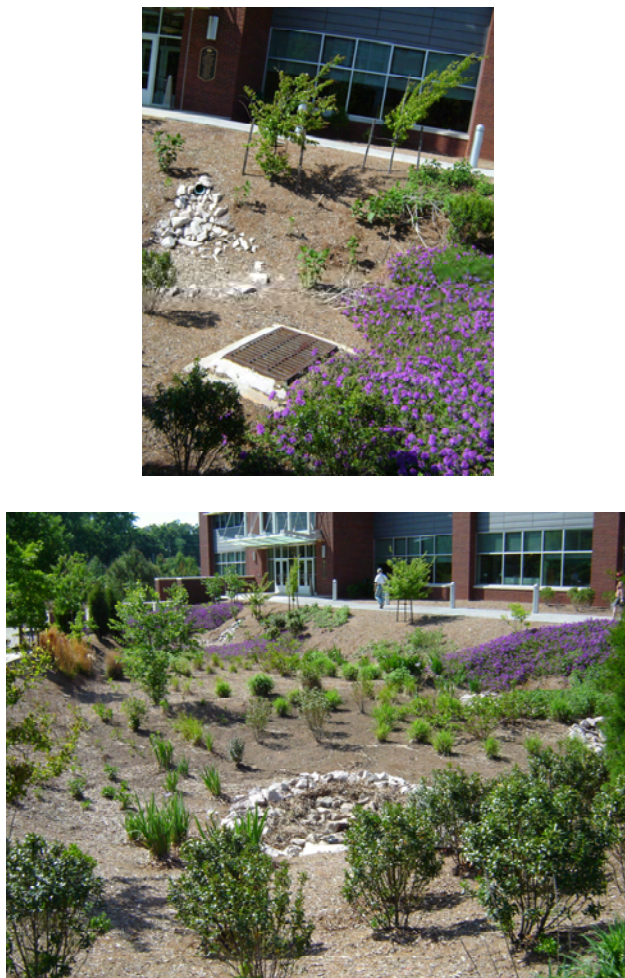
Figure 12-2c Bioretention Cell Without Pretreatment: Low-Sediment Influent
