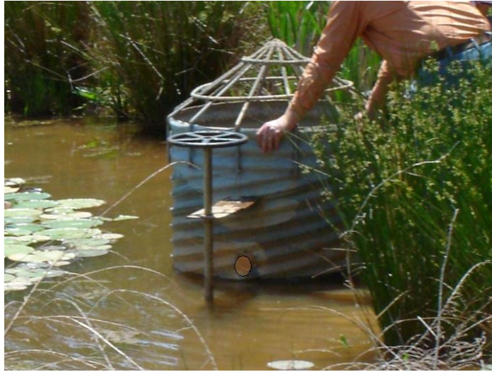
Figure 9-8 Outlet Structure With Manual Drawdown Valve for Maintenance
