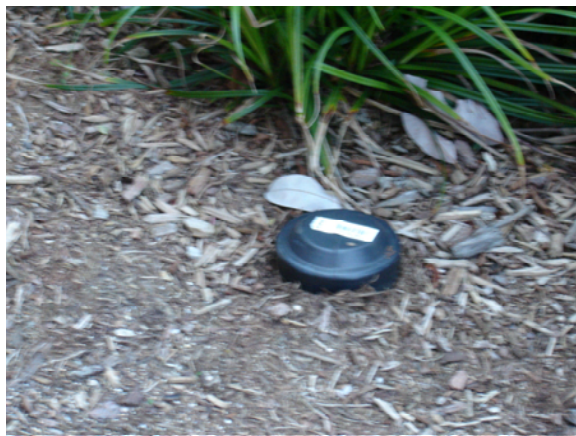
Figure 12-7 Bioretention Cell Clean Out Pipe
