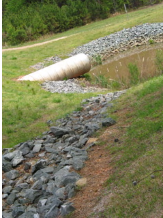
Figure 9-4 Wetland Inlet Device Examples: Culvert and Rip-Rap Channel (Courtesy of Sharon Schulze, NC State Science House)
