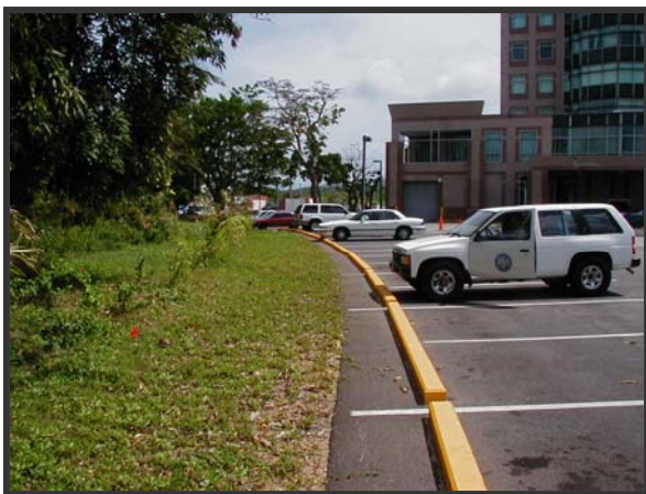
Figure 3.6 Use of a Grassed Filter Strip
