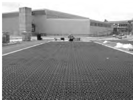
Figure 21.4 Permeable pavement: during and post construction
