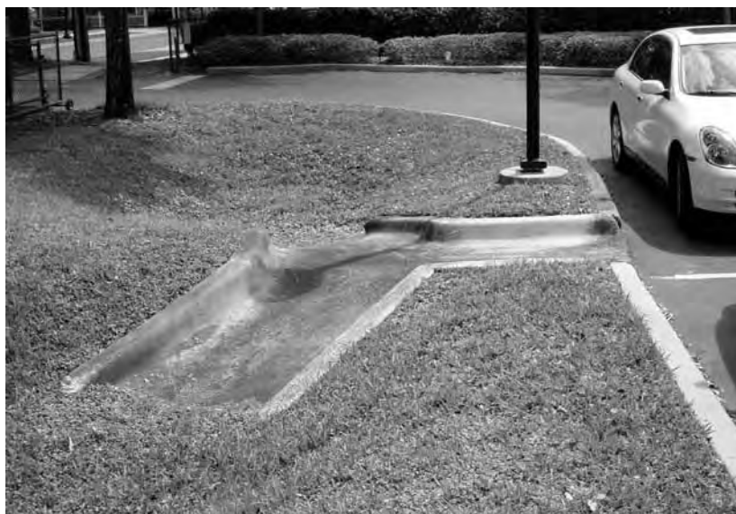
Figure 19.10 Alternative inlet bypass structure with low and high flow routes, Orlando, Florida, (courtesy Robert Bray Associates)
