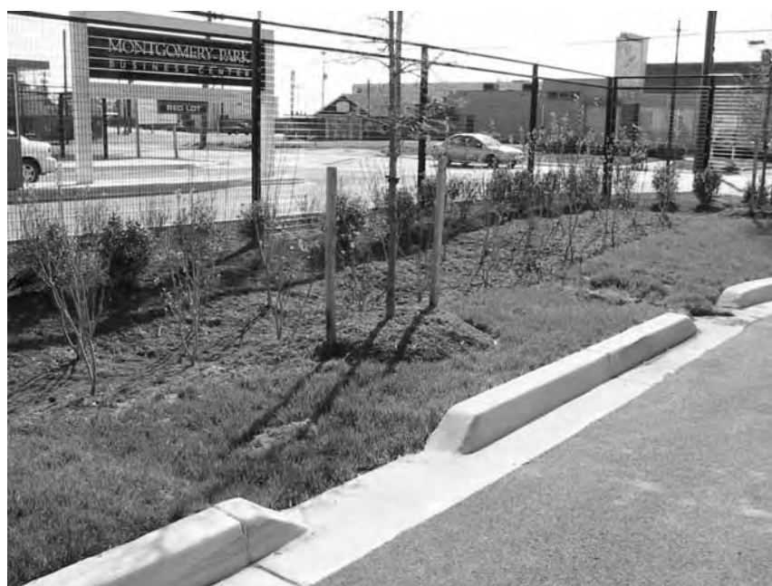
Figure 19.5 Roadside drop kerb lateral filter drain inlets (courtesy Robert Bray Associates)
