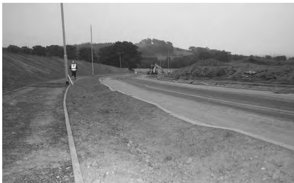
Figure 21.5 A swale under construction
