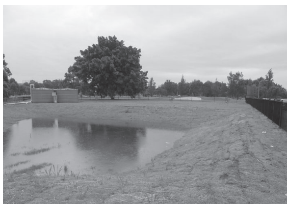
Figure 14.1 Surface sand filter
