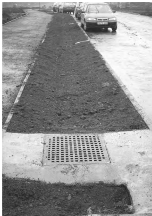
Figure 21.2 Construction of a swale
