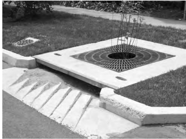
Figure 19.8 Highway inlet deflector system (courtesy Robert Bray Associates)
