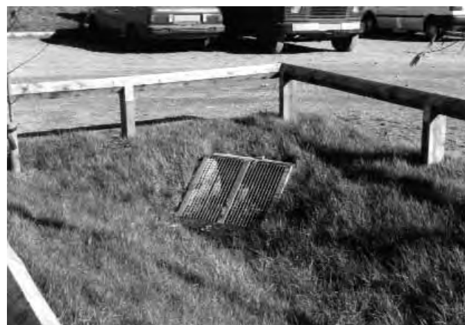
Figure 19.13 Photograph of screened orifice outfall with T-piece structure (courtesy Robert Bray Associates)
