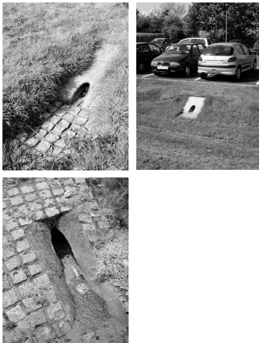
Figure 19.4 Photographs of low-flow inlet pipes to SUDS systems (courtesy Robert Bray Associates)
