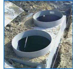
FIGURE 2 : SEPARATEUR A HYDROCARBURES [39]
