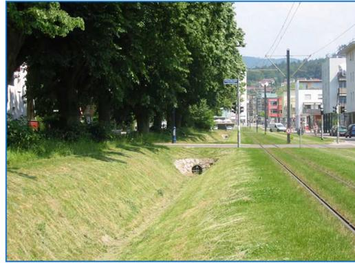
FIGURE 14 : NOUE (A GAUCHE) ET FOSSES D'INFILTRATION (A DROITE) EQUIPANT LE QUARTIER VAUBAN A FRIBOURG [64]
