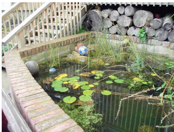
Small SUDS pool in high density housing – due to the close proximity to buildings hard edges are appropriate in this development, Stroud, Gloucestershire
