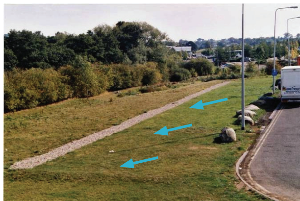
Filter drain protected from silt by a filter strip
