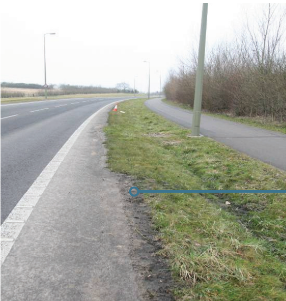
High grass at edge of road prevents water entering swale
