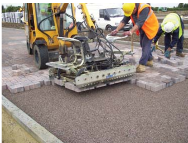
Permeable block paving being machine laid in Cambridgeshire
