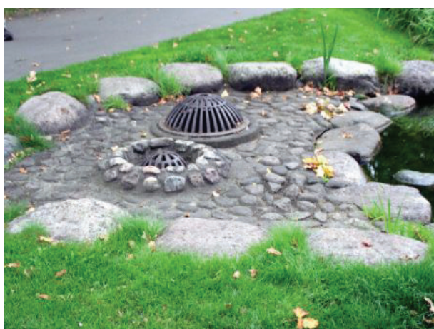
Overflow outlet from a pond
