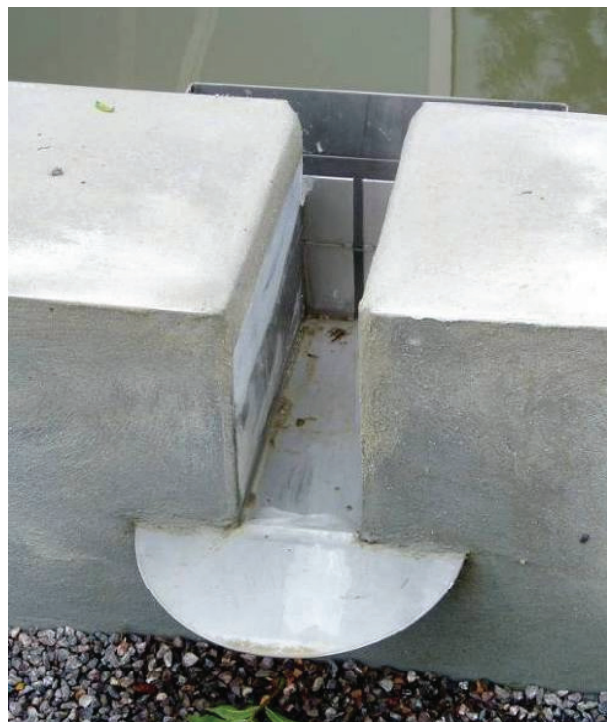
Slot weir outlet with steel plate to disperse water and debris guard behind
