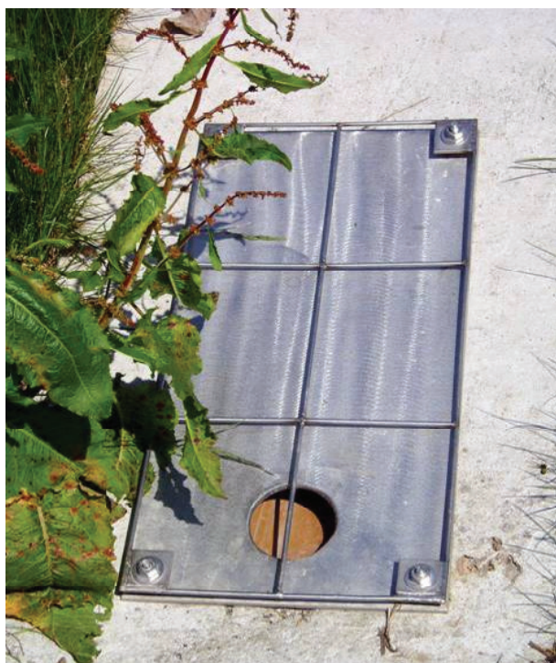
Orifice control to a basin located on the surface so that it is easily accessible
