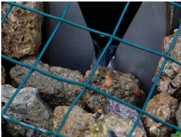
Recycled concrete used in a control structure in Cambourne, Cambridgeshire
