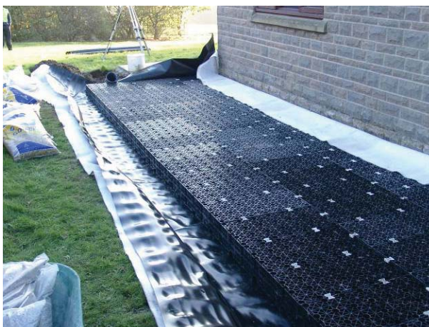
Rainwater harvesting tank being constructed below a patio, Derbyshire
