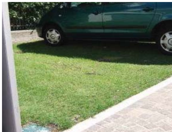
Reinforced grass car park surface, Lake Garda, Italy
