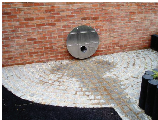
Stainless steel outlet leading to a surface rill
