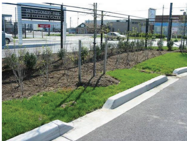
Dropped kerb inlet to rain garden
