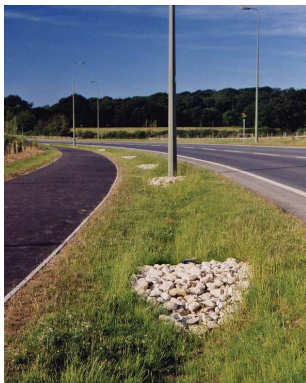
Shallow swale alongside a distributor road – check dams maximise storage and slow water, Witney, Oxfordshire
