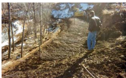
Photo 6. Construction of Brush Layering
