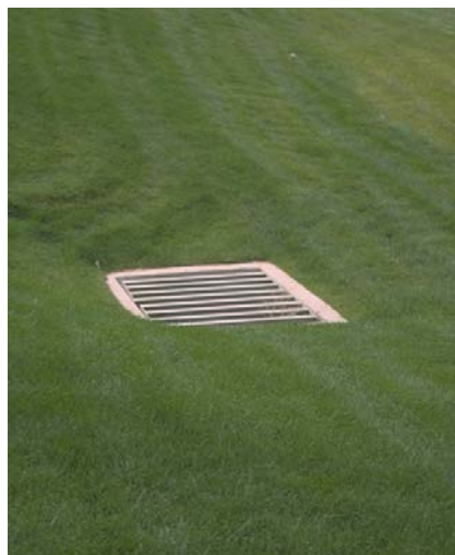
Photograph ST-6—Field inlets frequently need maintenance.
