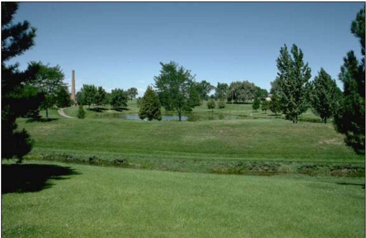
Photograph PL-2—A stable channel coupled with wet detention for the outlet of a large storm sewer system provides Denver enhanced water quality in Harvard Gulch.
