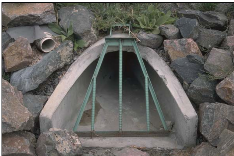
Photograph CU-6—Small trash racks at culvert entrance will increase the risk of entrance plugging.
