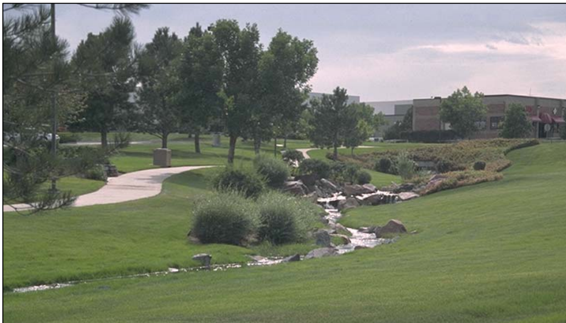
Photograph MD-6—Engineered grass-lined major drainageway with low-flow channel with bioengineered components integrated into the design.
