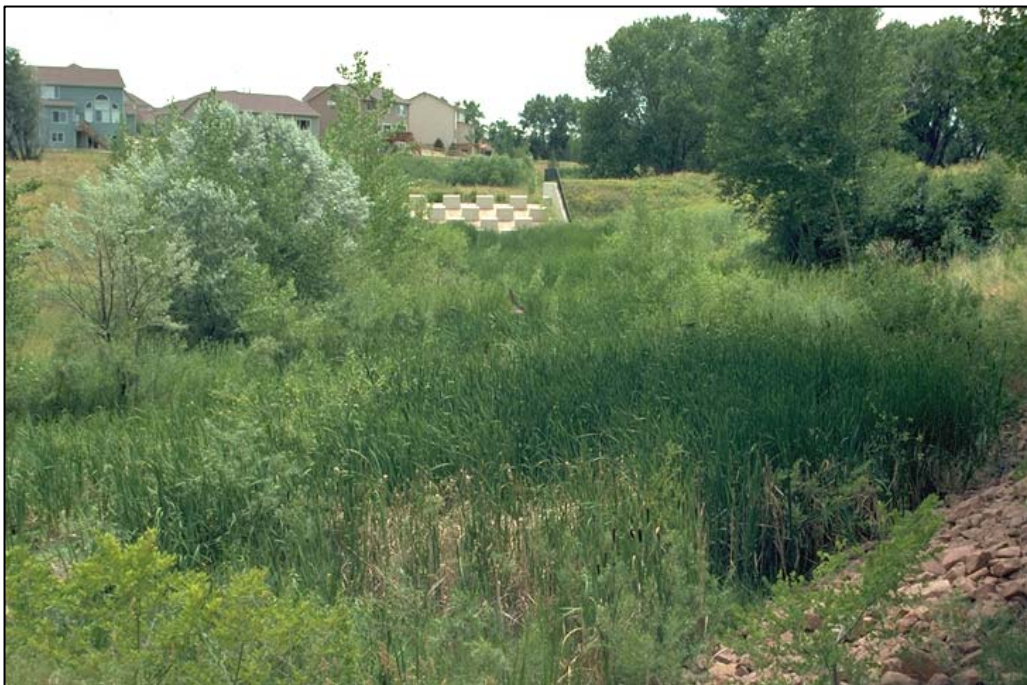
Photograph MD-11—Bioengineered major drainageway with dense and diverse vegetation and energy dissipator.
