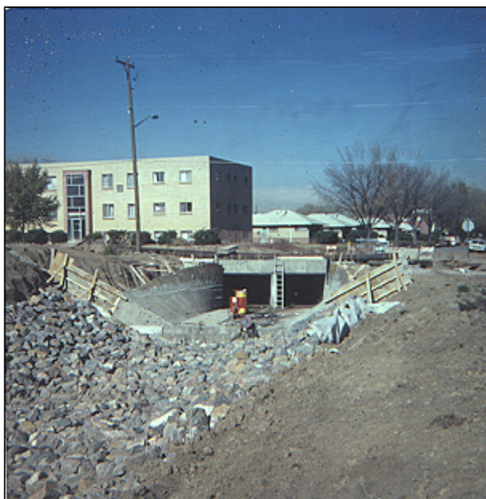
Photograph MD-9—Riprap channel. Burying and revegetation of the rock (i.e., soil riprap) could make this site blend into the adjacent terrain very nicely.
