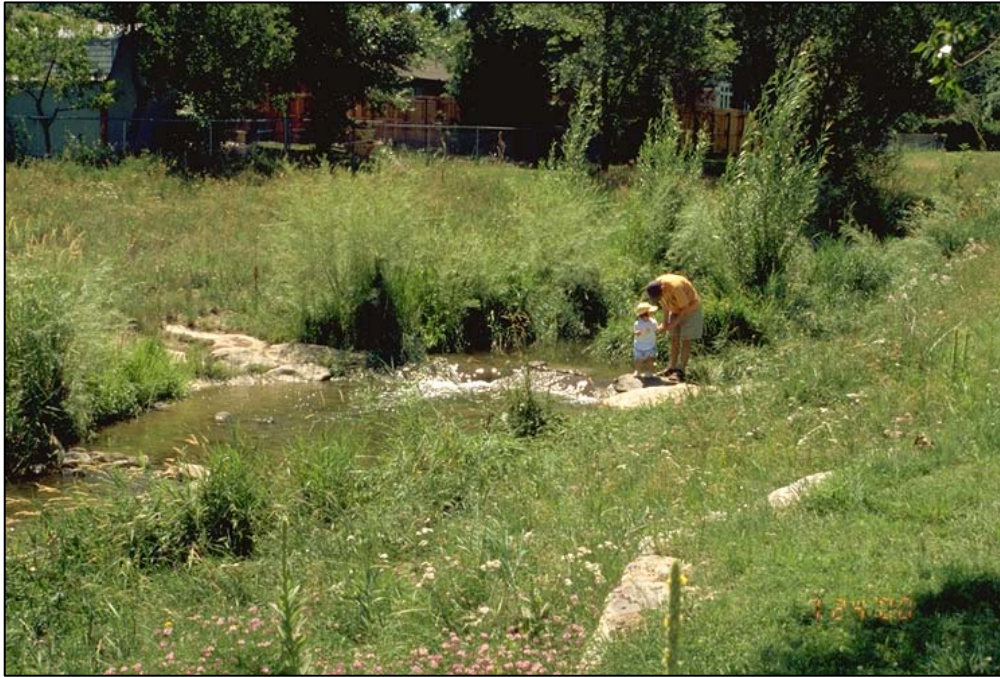
Photograph MD-10—Bioengineered major drainage channel using low-grade control structure provides long-term structural integrity and diverse ecology.
