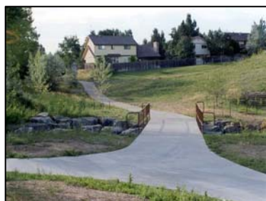
Photo 3. New Grouted Boulder Structure & Pedestrian Bridge
