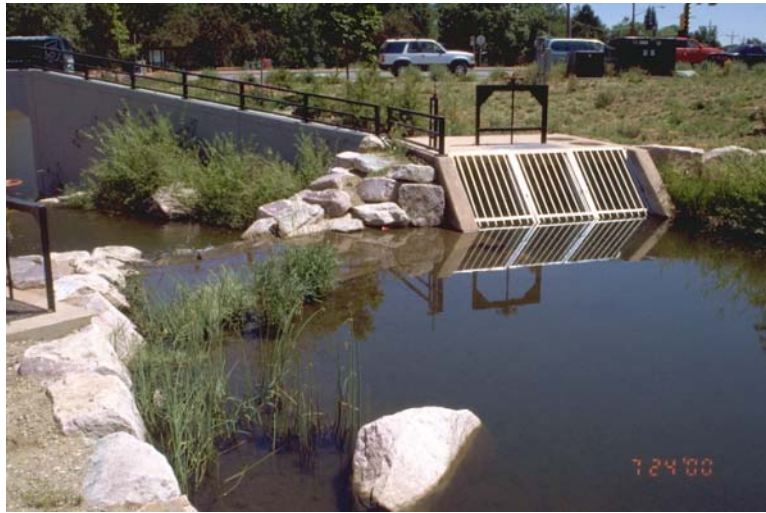
Photograph CU-4—Public safety features such as the rack at the entrance to an irrigation ditch and the railing on the wingwalls must be considered.
