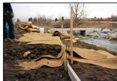
Photo 9. Construction of Wrapped Soil Lifts
