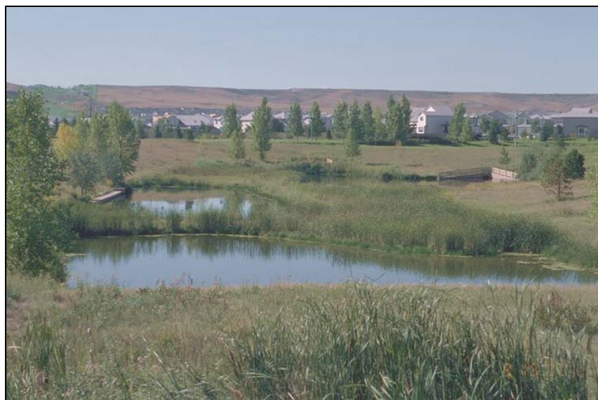
Photograph MD-13—Integration of open water areas with major drainageways provides habitat and aesthetic benefits in addition to providing storage.
