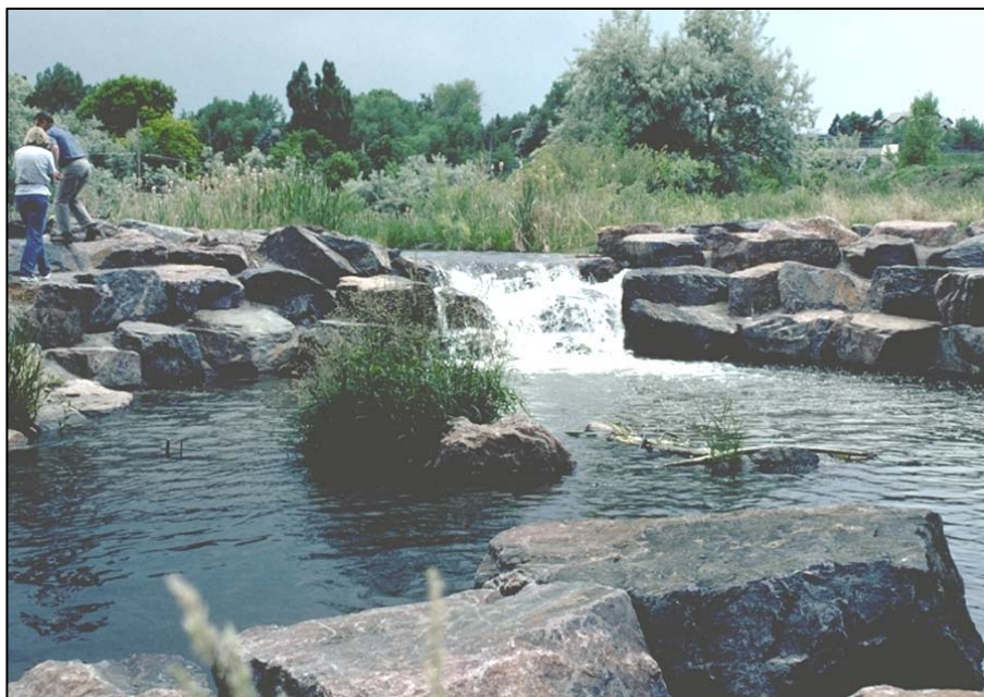
Photograph HS-6—Detail of the grouted sloping boulder drop with a trickle channel section creating the sight and sound of cascading water.
