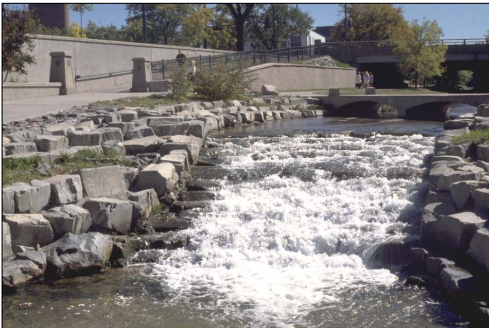
Photograph HS-5—Example of stepped downstream face for a sloping boulder drop structure. Note dissipation of energy at each step for low flow.
