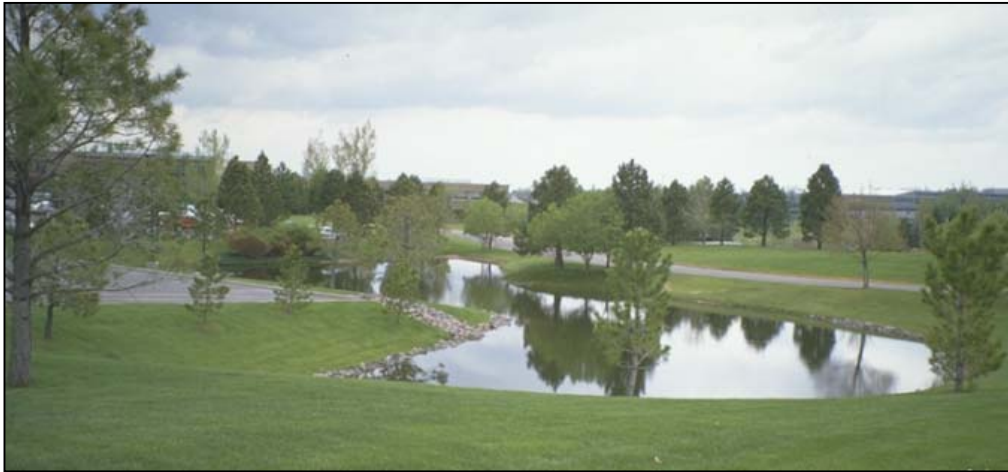
Photograph DP-5—Detention basins with permanent ponding help in many ways, including flood reduction, water quality and land values.
