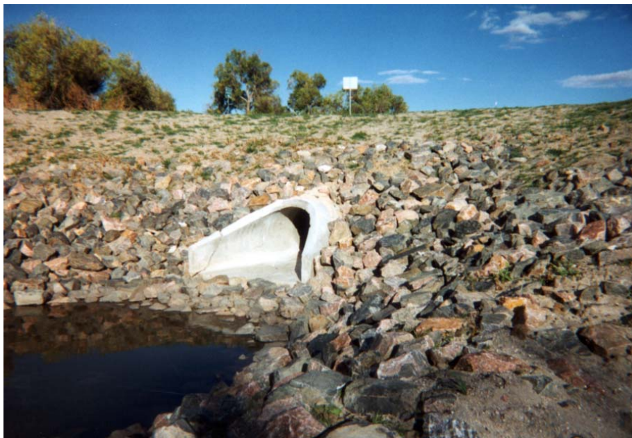
Photograph HS-13—Culvert outlets when left unprotected cause downstream erosion. The designer's job is not complete until provisions are made to protect the outlet. Use of vegetated soil-riprap would blend this structure better into the natural landscape.
