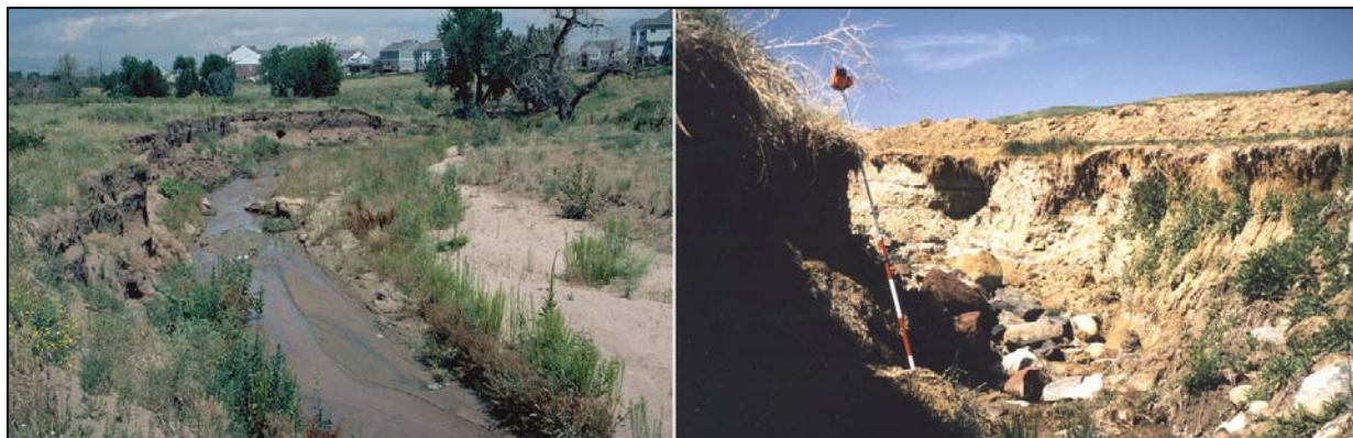
Photograph MD-4—Channel degradation in an unstable channel.
