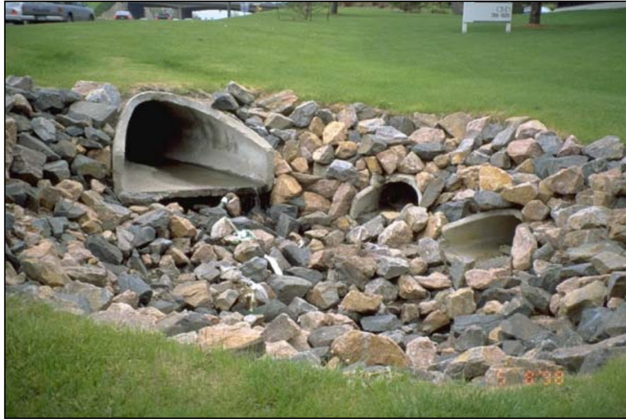
Photograph CU-5—Energy dissipation and outlet protection are essential to promote channel stability.
