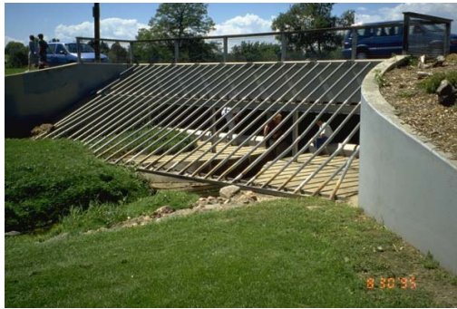
Photograph CU-1—Public safety considerations for long culverts should be accounted for with culvert designs such as with this collapsible trash rack at a park-like location.
