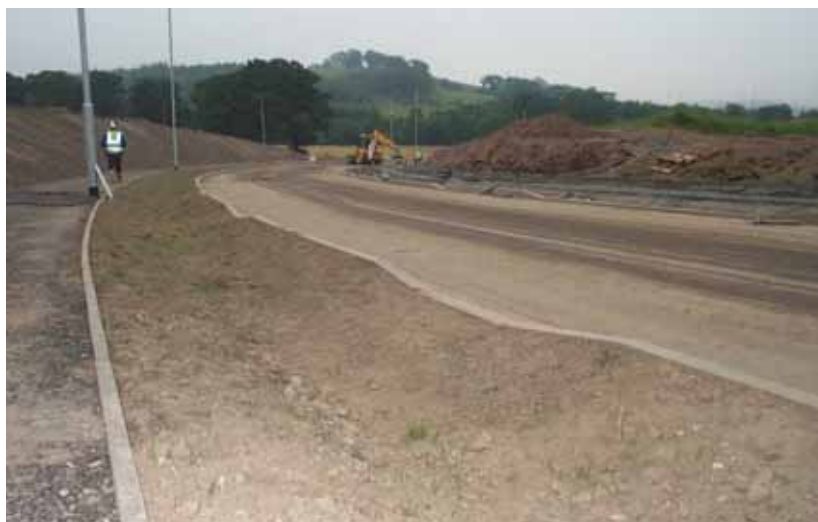
Figure 11.6 A swale under construction
