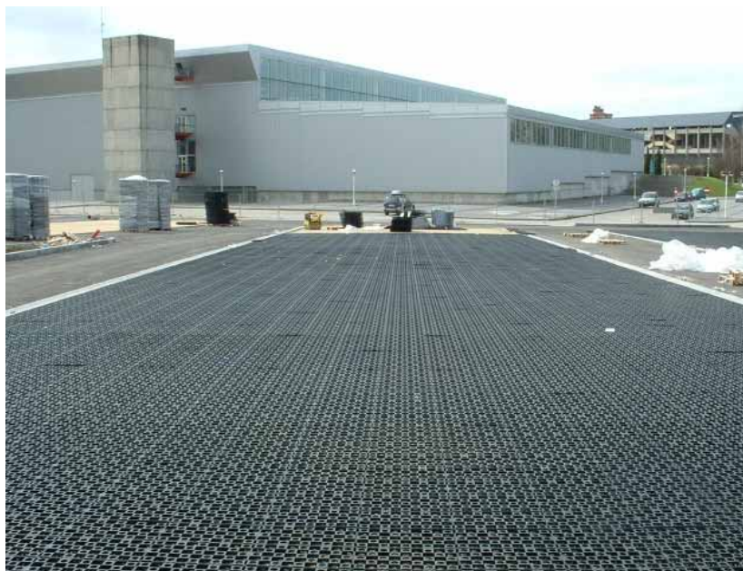
Figure 11.9 Example of proprietary geocellular system under construction
