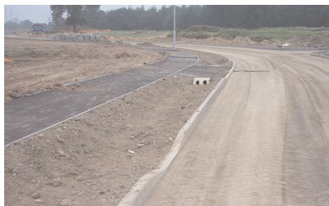
Figure 7.1 Construction of a swale
