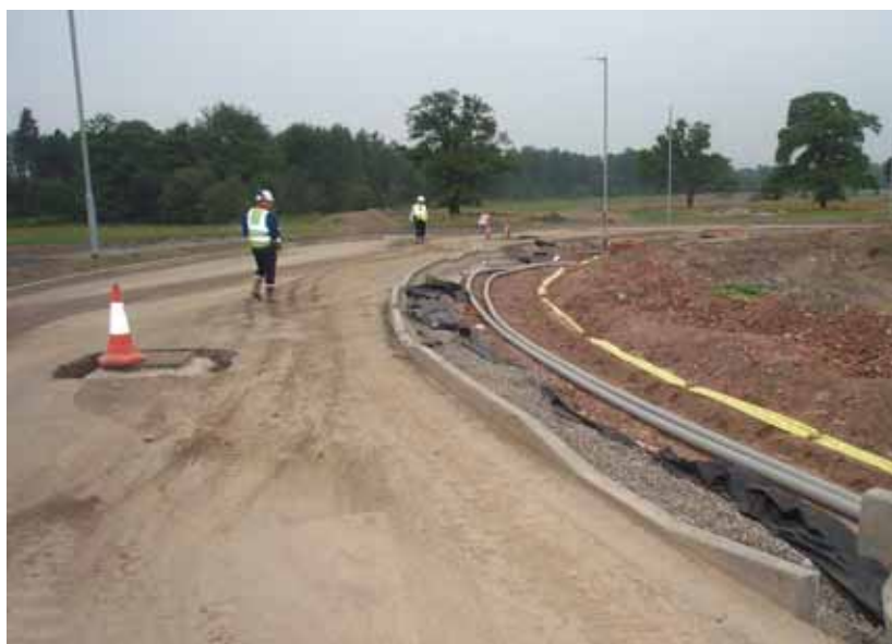
Figure 11.5 A filter trench under construction
