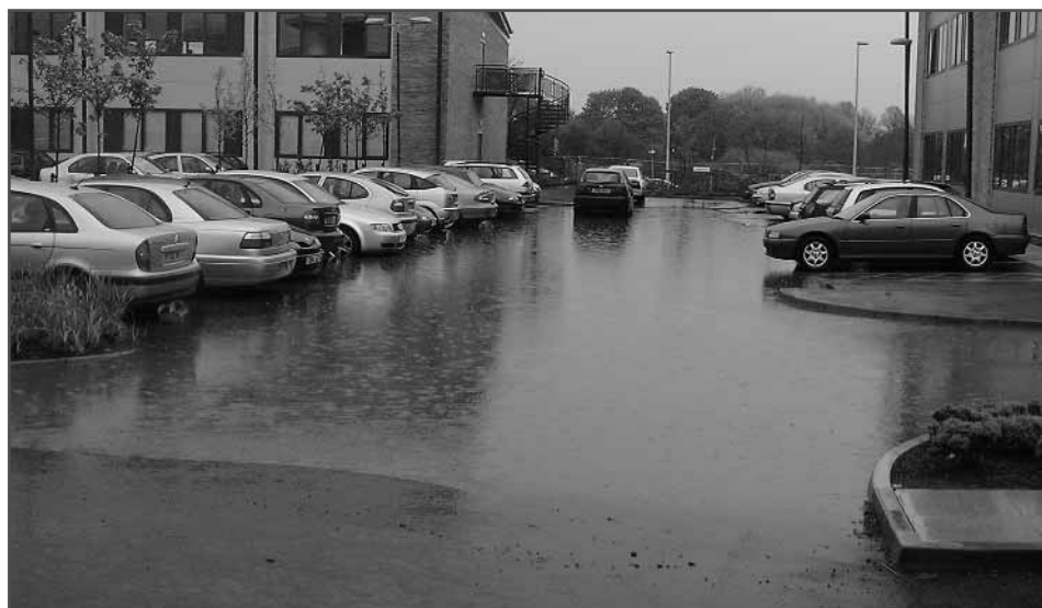
Figure 12.7 Temporary ponding in car park showing the storage potential during an extreme event
