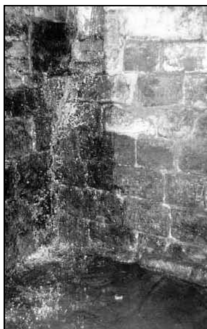
Figure 5.4 Cellar flooding from infiltration from a local watercourse
