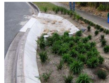
Dense vegetation downstream of inlet can assist with the capture of sediment
