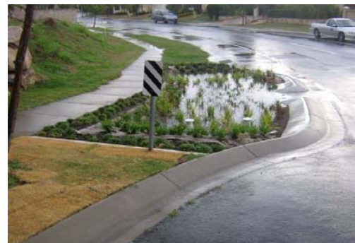
A stormwater garden retrofitted into an established residential area of Brisbane
