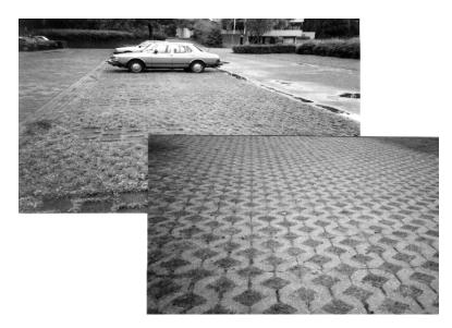
(a): Example of block-reinforced grass used for vehicle hard-standing areas
