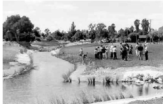
*Figure 24b. Bannister Creek post-engineering (restoration) works summer 2001. The channel was realigned to create a winding creek and the banks reshaped to a gentle slope and stabilised. (Photograph: Department of Environment.)*
