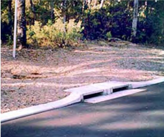
Figure 3. Side entry pit and bubble-up located within mulched detention area. (Photograph: TME 2003.)
