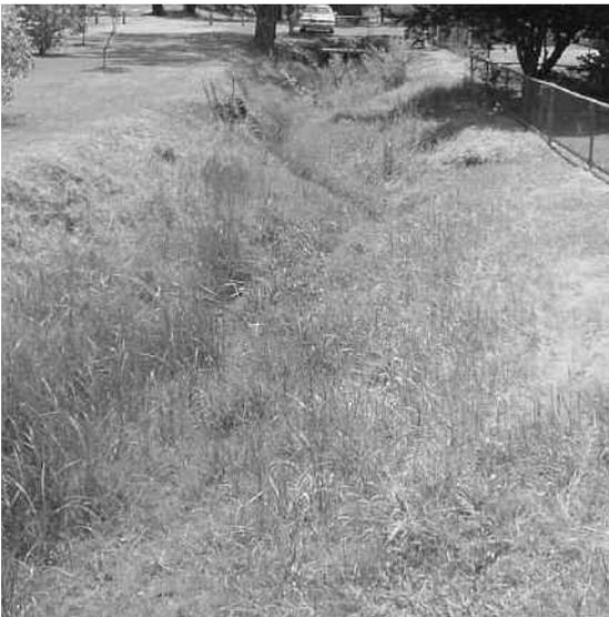
*Figure 14a. Geegelup Brook, Bridgetown, before restoration works – a weed infested trapezoidal drain. (Photograph: Department of Environment, 2003.)*
