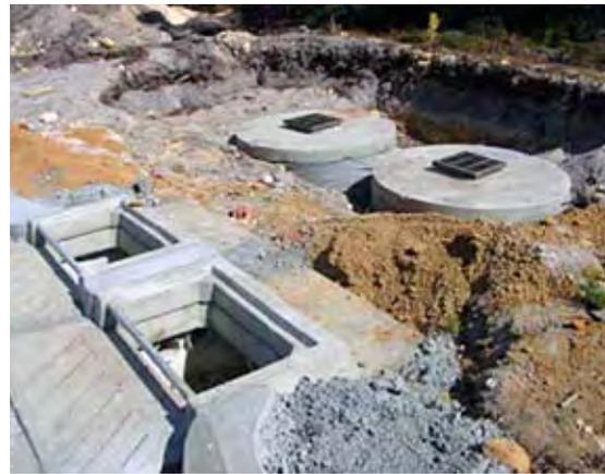
Figure 6. Construction of side entry pits to capture road runoff and divert it into soakwells that have bubble-up lids and are located within a detention area. (Photograph: TME 2003.)
