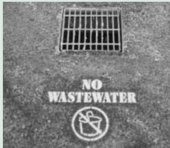
Figure 1. Industrial site drain stencil. (Photograph: Colin Ceresa, ARRIX.)
