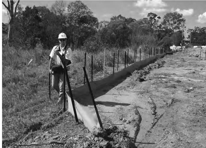
Figure 5. Silt fence for controlling sediment during land development. (Photograph: André Taylor, Ecological Engineering Pty Ltd.)
