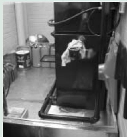
Figure 1. Green Stamp automotive premises, Balcatta. Correct storage of fuel and other chemicals in a bunded area. (Photograph: Department of Environment.)
