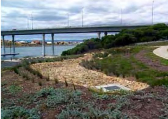
*Figure 1. Bioretention swale, soon after construction and planting in Dawesville. (Photograph: Grahame Heal, City of Mandurah, 2006.)*
