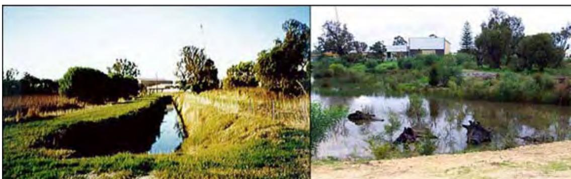
*Figure 7. Black Creek trapezoidal drain converted to a constructed wetland, City of Cannington. (Photographs: (left) JDA 1999, (right) Water and Rivers Commission 2003.)*
