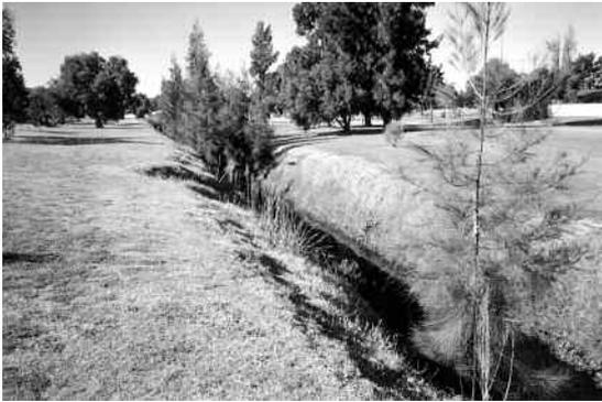
*Figure 24a. Bannister Creek before restoration works (1999) – a straight trapezoidal drain with steep grassed banks and high velocity flows. (Photograph: Department of Environment.)*
