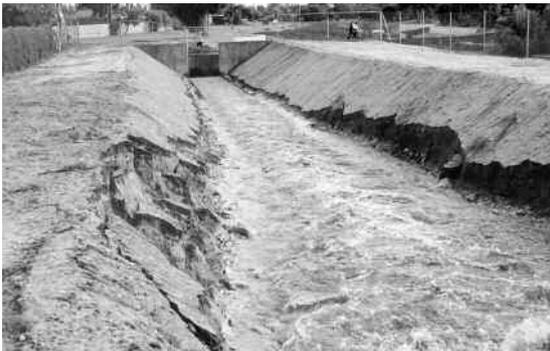
*Figure 25a. Flood damage of the trapezoidal drain upstream of the rehabilitation reach of Bannister Creek. (Photograph: Department of Environment.)*
