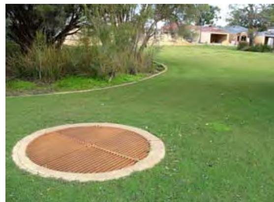
Figure 3. Bubble-up pit located in a park. (Photograph: Department of Water 2006.)
