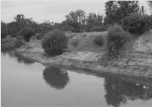
*Figure 1. Sediment excavated from the Harvey Main Drain and stockpiled on the banks. Sediment has buried fringing vegetation and may be washed into the waterway. (Photograph: Department of Environment.)*
