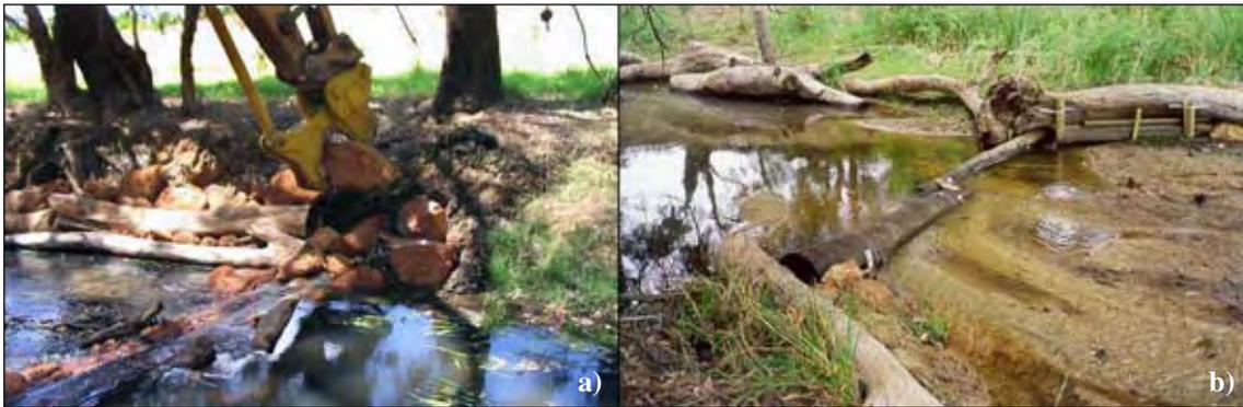
Figure 5. a) Construction of a log and rock riffle structure in the Canning River, Pioneer Park, Gosnells. (Photograph: Department of Water 2004.) b) Log riffle built on the South Dandalup River, Pinjarra, to stabilise the sandy riverbed, induce a scour pool and enhance habitat diversity. (Photograph: Water and Rivers Commission 1999.)
