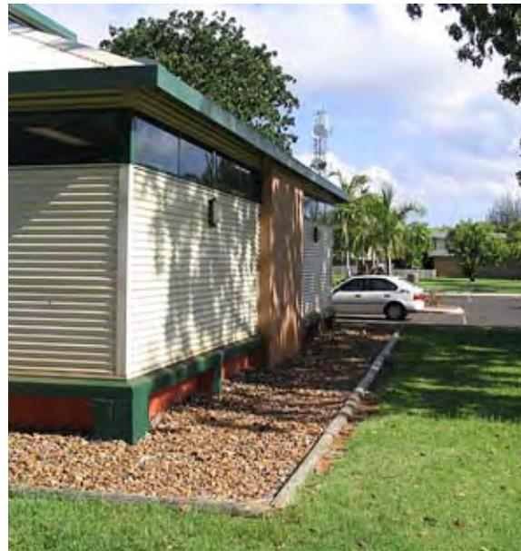
*Pervious surface under gutterless roof, Shire of Broome. (Photograph: Allan Ralph, Shire of Broome 2005.)*
