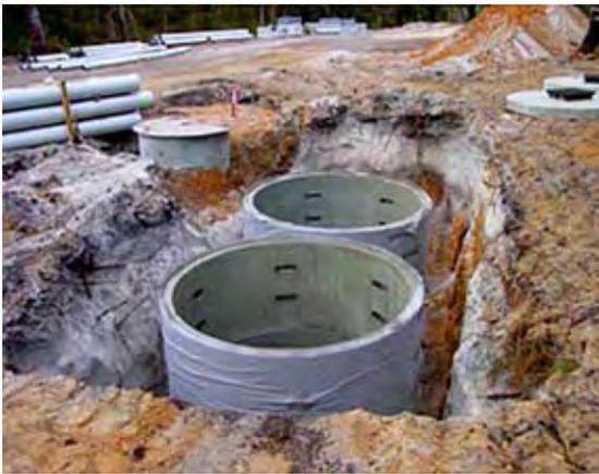
Figure 5. Soakwell construction. (Photograph: TME 2003.)
