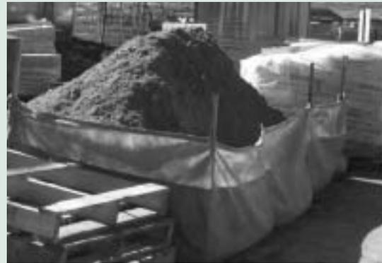
Figure 6. Soil stockpile contained by a sediment fence. (Photograph: Clean Site, Keep Australia Beautiful Council WA.)
