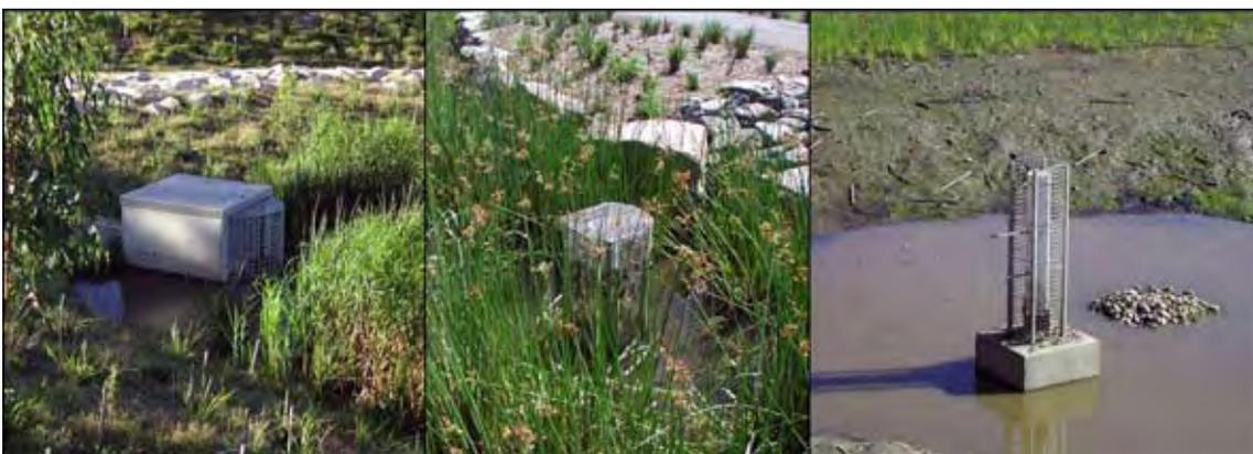
Figure 6. Debris guard examples for riser outlets. (Source: Morton Bay Waterways & Catchments Partnership 2006.)
