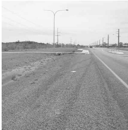
*Figure 10. Example of a kerbless road and swale, Dampier Road, Karratha. (Photograph: Department of Environment, 2006.)*
