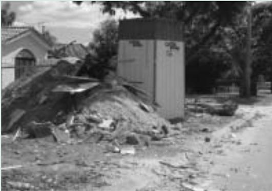
*Figure 1. Inadequate waste containment and spillage of waste onto the road. (Photograph: Clean Site, Keep Australia Beautiful Council WA.)*
