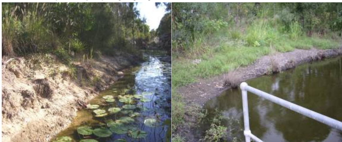
Figure 5-2 Examples of Erosion within Constructed Wetlands
