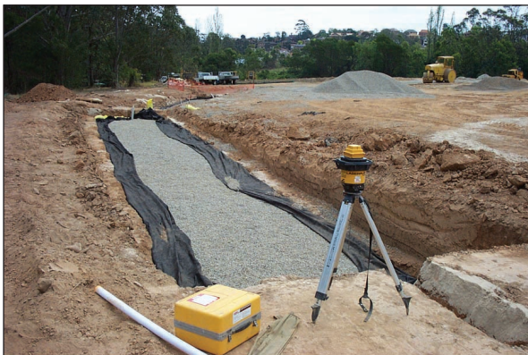
The completed tank covered with free draining material
