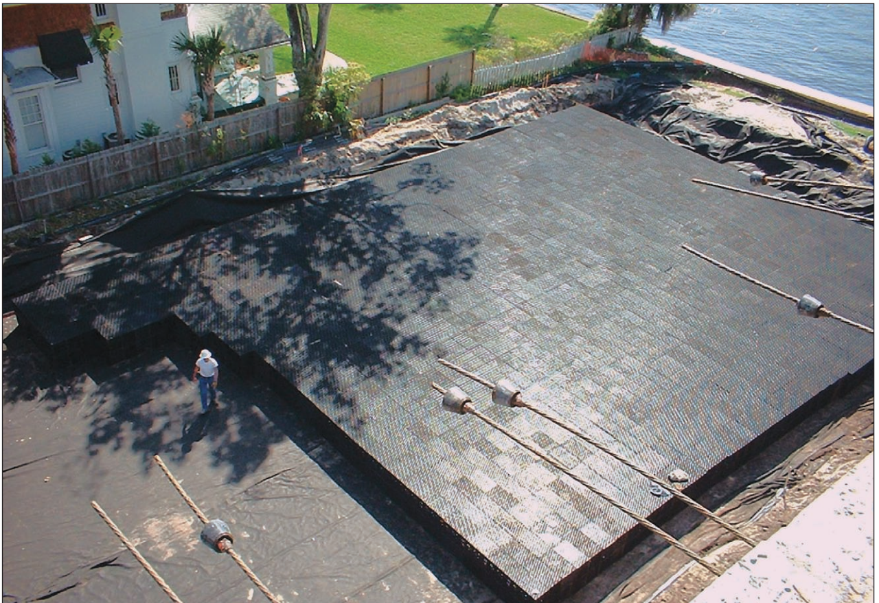
Installation of the Matrix® tank modules
