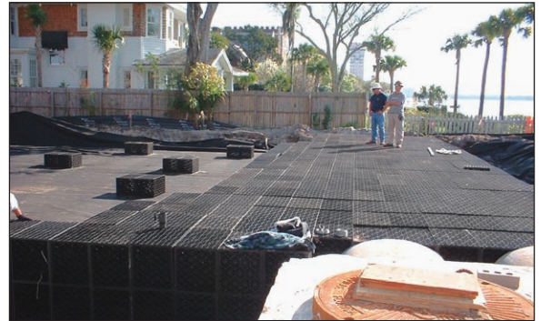
Installation of the Matrix® tank modules
