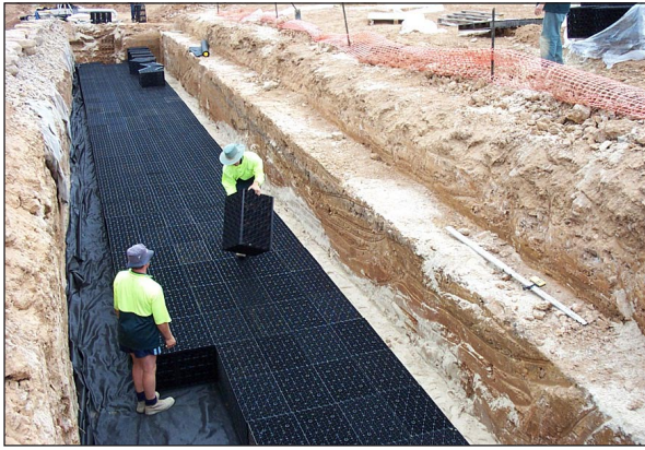
Installing the tank modules
