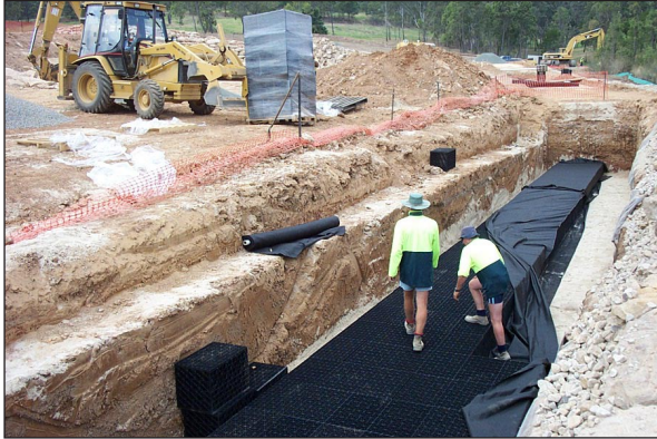
Wrapping the tank in Geotextile
