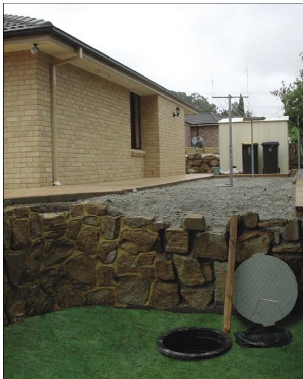
An Atlantis® Filtration Unit installed into the garden area.
