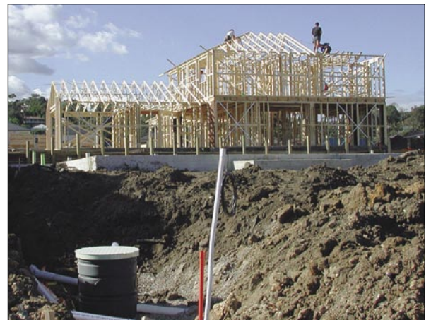
Installation of an Atlantis® Filtration Unit in the garden area of new home.
